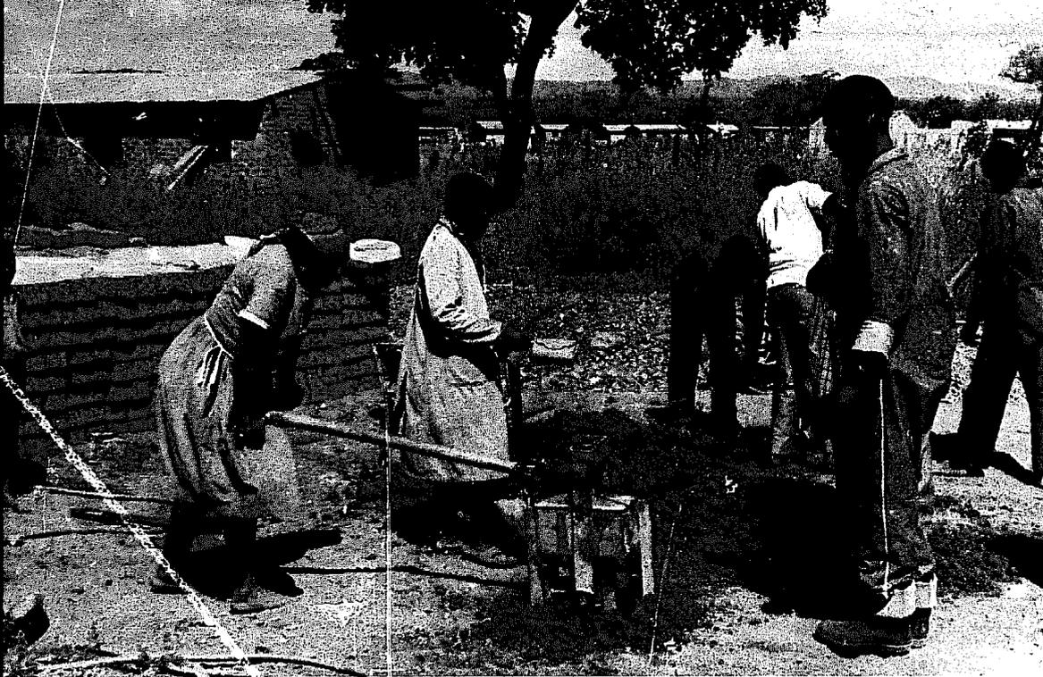
Pressing the earth and cement mixture in the Cinva-Ram which produced the bricks.
