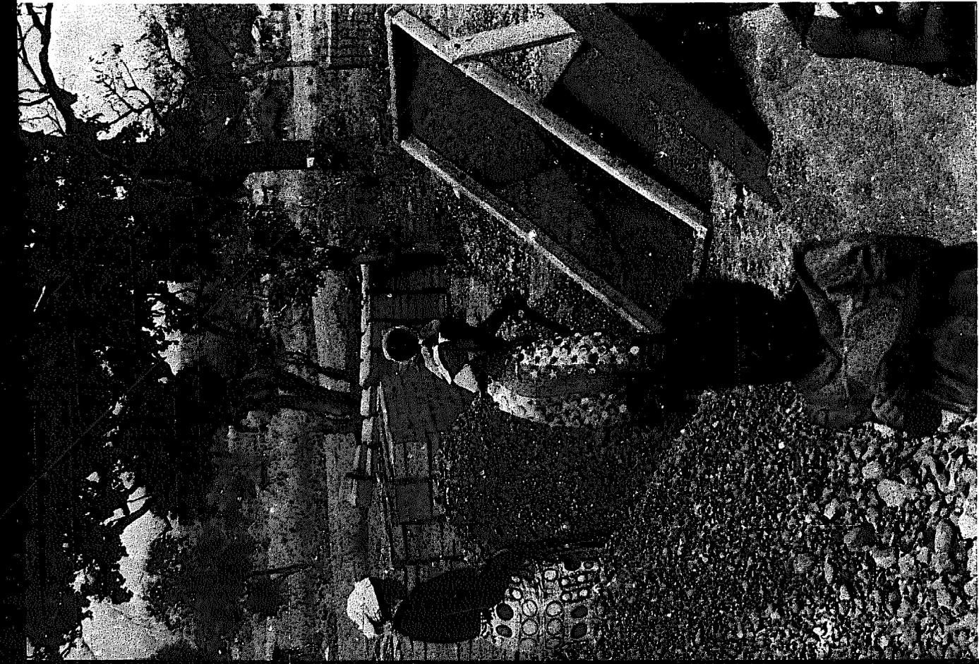
Sieving separated the fine earth for brick-making from the coarse material that was used to fill in under the floor.
