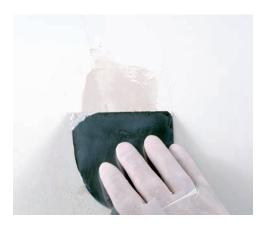
**3.** Wipe the broad knife downward over the crack to remove excess compound, and then let the layer dry thoroughly.
