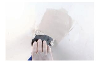
**4.** Repeat Step 3 two more times or until the patch is level with the wall, taking care to keep each layer thin.
