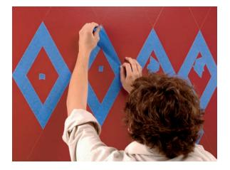
**5.** Starting with the row closest to the ceiling, apply blue painter's tape to the penciled lines on either side of the diamonds marked in Step 4. Tape off all the diamonds in this row, and *burnish* the tape by running a plastic putty knife or credit card over it in both directions to make sure the tape is pressed tightly against the wall and the paint won't bleed under it.
