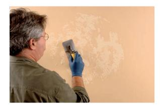
**3.** Put on latex gloves, and use the steel trowel to apply plaster in a thin coat. Start in a corner, and use long and short strokes that crisscross over each other at varying angles. Don't worry about covering the entire wall; leaving small bare spots as you apply the first coat is preferable.
