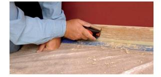
**3.** If water has raised the grain of the wood underneath (you can tell because the wood will be bumpy), take off enough paint to expose adjacent undamaged wood. Use 180-grit sandpaper to sand the damaged spot until the wood itself is smooth.
