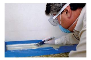
2. Read the directions on the container of chemical stripper that you've selected to use. Following the product directions, use an old paintbrush to apply the stripper to the surface of painted trim. Work in a small section of trim to get a feel for the amount of time it takes for the paint to lift and peel off easily; you can increase the size of the section as you proceed around the room.
