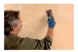
7. Wearing gloves, apply a second thin coat of plaster by using the steel trowel and the same crisscross technique. Make sure you cover the entire wall, leaving no gaps or low spots.
