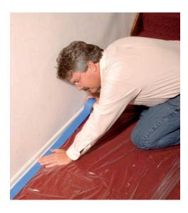
**3.** Cover the floor with one or more plastic dropcloths. Tape it down with blue painter's tape to avoid slippage.
