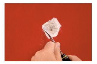
**2.** Scrape damaged and loose plaster away from the hole with the tip of a screwdriver.
