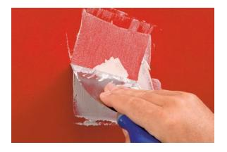
**4.** Using a broad knife, fill the crack or hole with the patching compound, and smooth the compound with the flat edge of your knife. (A broad knife works better than a wide-blade putty knife because its sharp edge removes excess plaster and smoothes the patch better.)
