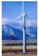
A horizontal axis turbine. Courtesy Vision Quest Wind Electric Inc.
