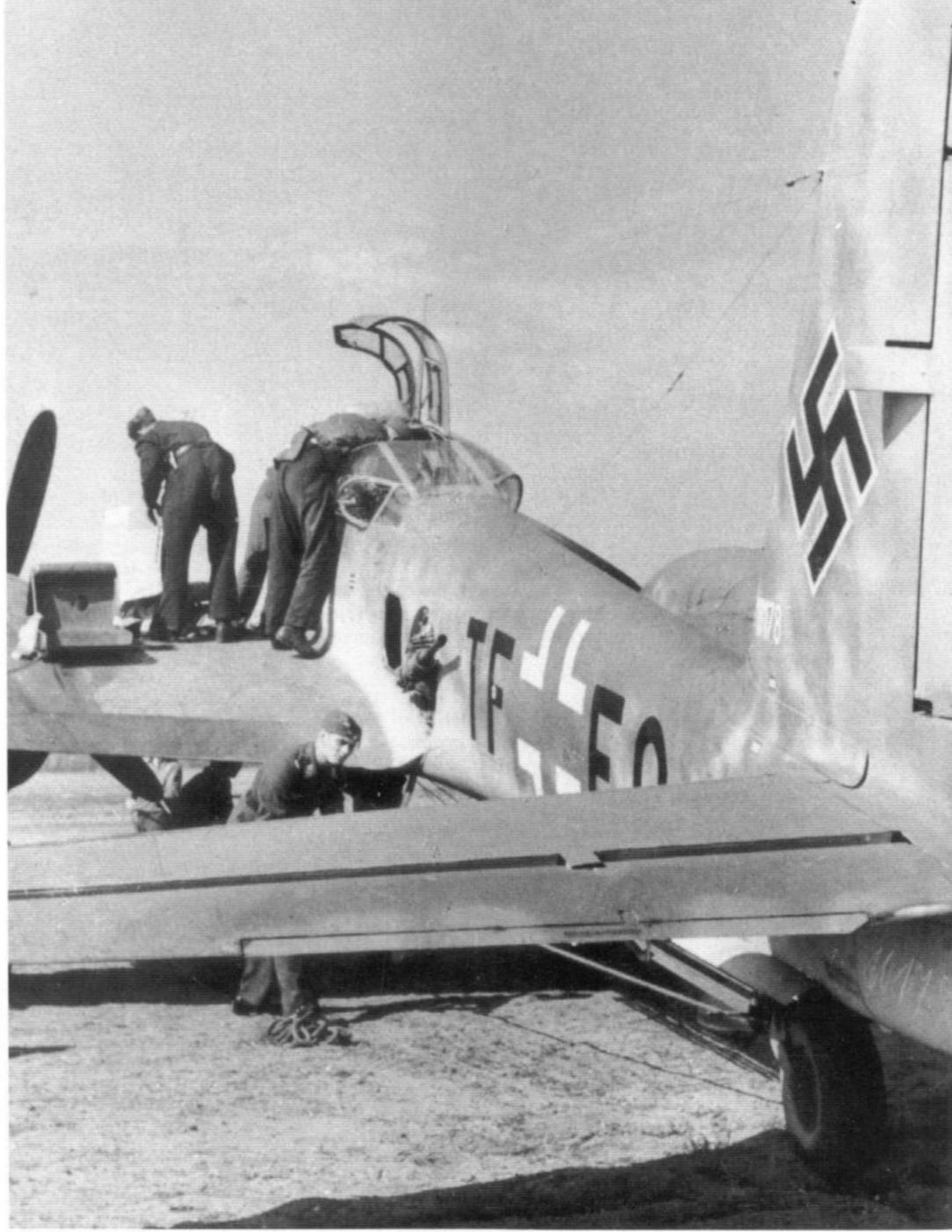
Ground crewmen service a Me 410B-1 (TF+EQ) stationed in Le Mans, France. The aircraft was part of Stab/3.Jagd-Division. The covers over the 13mm side gun mounts have been removed so that the guns can be serviced and reloaded. (Dressel)
