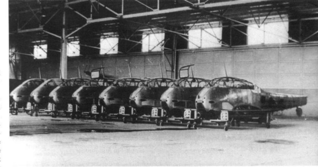
Early production Me 210 fuselages rest on four wheel dollies in the Messerschmitt work shop. These aircraft were fitted with the early style cockpit canopy. While the side turret mounts are in place, the 13mm guns have not been mounted. (Mohr)
