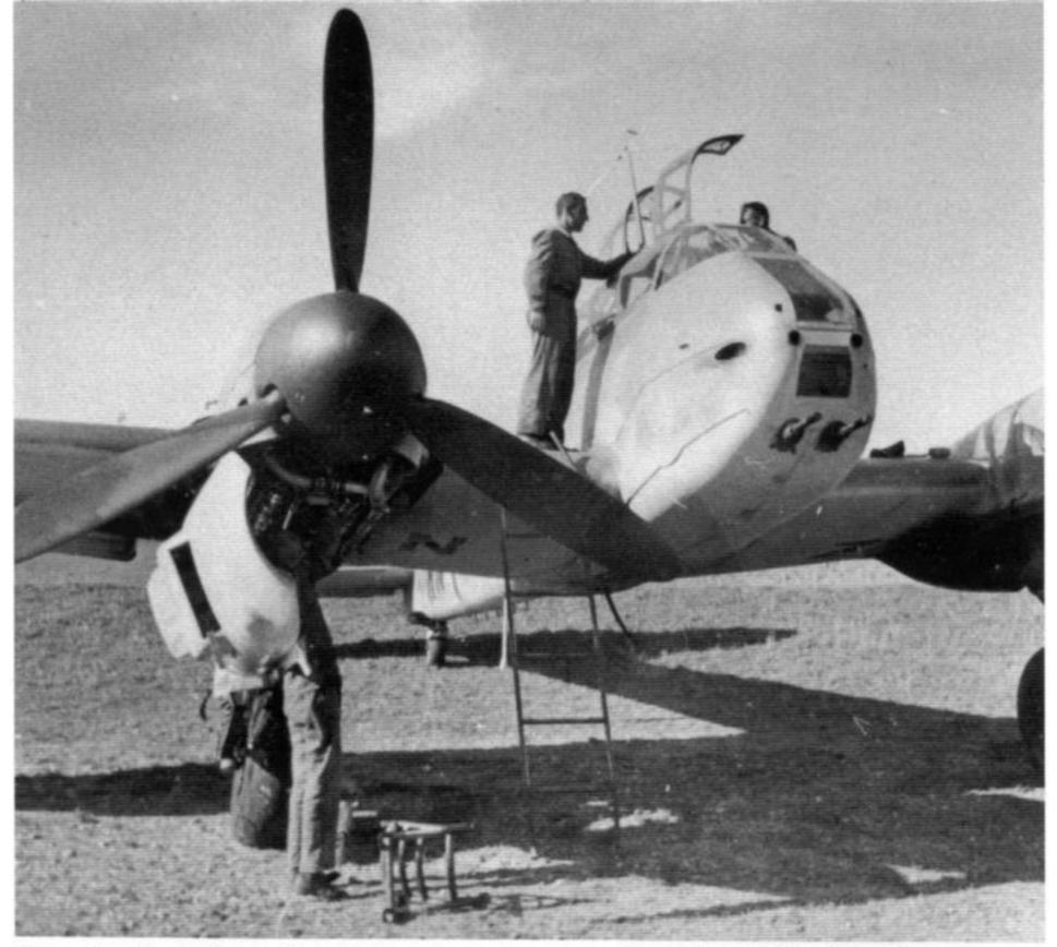
A mechanic works on the starboard engine of an Me 410B-2/U2/R2 (RN+Z) during the summer of 1944. In addition to its standard armament, the aircraft carries two additional MG 151 20mm cannon in the weapons bay. (Radinger)
