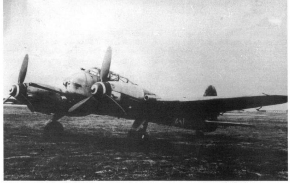
This Me 410B-2/U-4 armed with a 50mm BK-5 cannon was captured and evaluated by the Soviets. The aircraft was tested at Ramenskoye airfield in Moscow during 1945 and was only partially repainted with Soviet insignia. (Gretzyngier)
