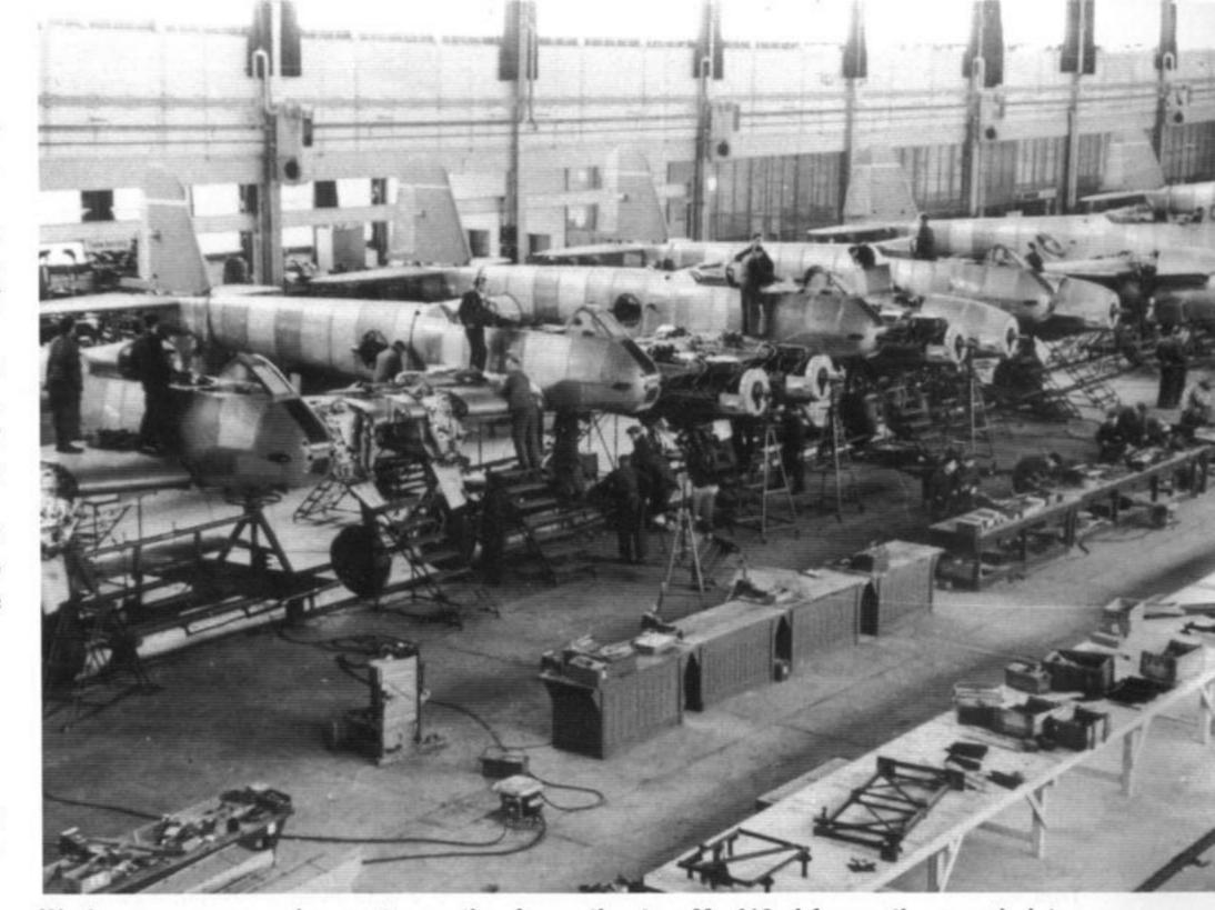
Workmen prepare a wing center section for mating to a Me 410 airframe, the round plates on the wing are service access panels.. The airframes in the background have their center sections in place along with the main landing gear. (Stapfer)
