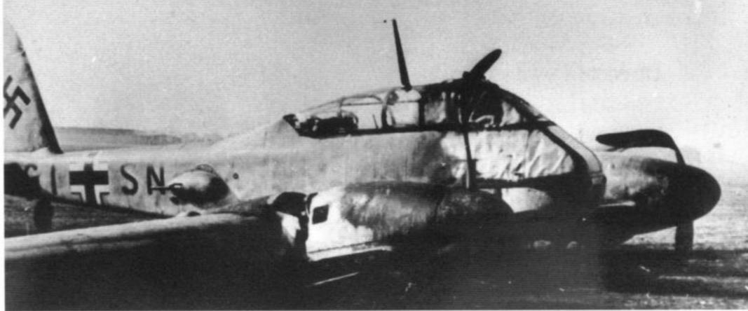
The Messerschmitt Me 210 program was plagued with accidents. The Me 210V-10 prototype (GI+SN Werk Nr. 010) ended up on its belly after the landing gear failed on landing after a test flight on 16 June 1941. (Mohr)
