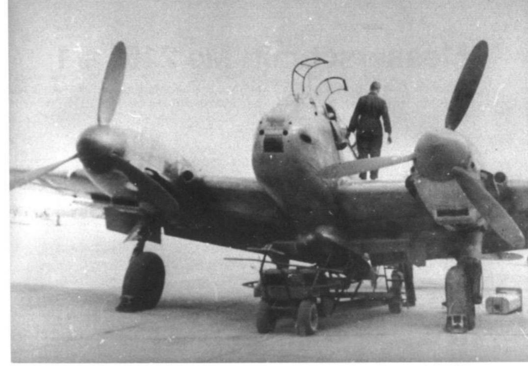
This Me 210 (DI+NF, Werk Nr. 0194) has an L 10 glider and LT 950 torpedo mounted under the fuselage at the Luftwaffe test base at Gotenhafen, Hexengrund, during June of 1942. (Nowarra)
