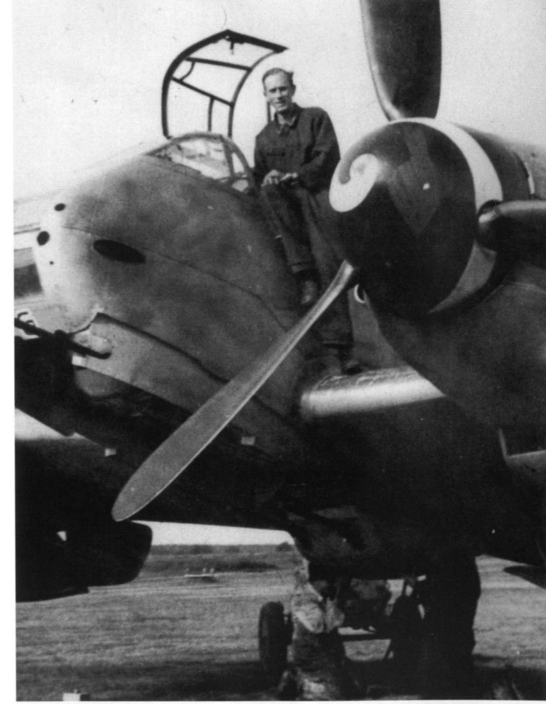
A Me 410B-1/U2 outfitted with a R4 container (two MG 151 20mm cannons) under the fuselage on the airfield at Konigsberg-Neumark during the Summer of 1944. The aircraft has the individual aircraft number, 6, on the nose in Black with a thin White outline. (Petrick)
