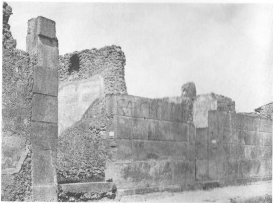
Figure 3 Façades of upper-class houses in region VI. The façades of these houses from the second century B.C. can still be easily recognized today by their walls of neatly hewn tufa blocks. The entrances often have carved door frames, sometimes with elaborately sculpted capitals (compare figs. 6 and 7).
