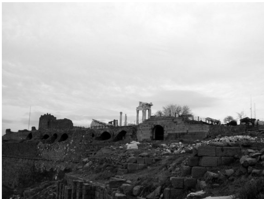
Fig. 2. Vaulted chambers supporting the Trajaneum platform.
