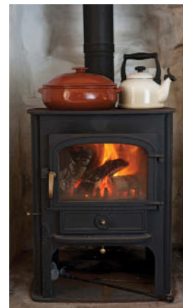
Fig. 7.1.1 This wood-stove transfers heat to the room by conduction through its metal walls, convection of air past its surfaces, and radiation from its black exterior.
