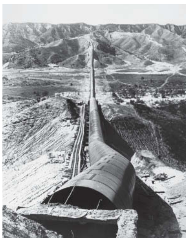
Fig. 5.2.6 Los Angeles receives much of its water from Owens Valley, 300 km to the north. The water negotiates the mountains and valleys in between, driven by gravity alone. Giant pipes allow pressure to build during downhill stretches to push the water back uphill later on. Parts of the 1913 aqueduct support so much pressure that the steel pipe used in them has to be more than an inch thick.
