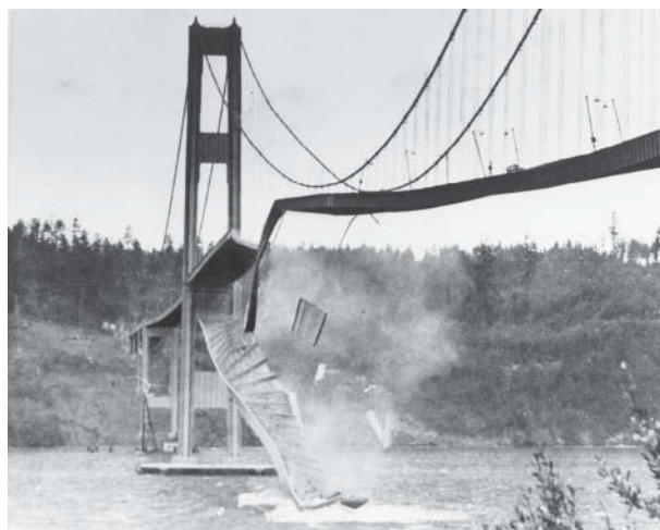
Fig. 9.2.7 The Tacoma Narrows Bridge collapsed in November 1940, as the result of resonant energy transfer between the wind and the bridge surface. Shortly after its construction, the automobile bridge began to exhibit an unusual natural resonance in which its surface twisted slowly back and forth so that one lane rose as the other fell. During a storm, the wind slowly added energy to this resonance until the bridge ripped itself apart.
