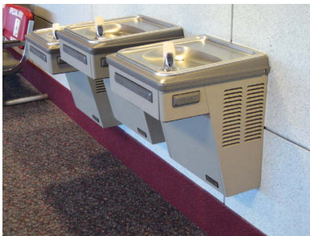
Fig. 8.1.8 These drinking fountains have heat pumps built into them to cool the water. Heat removed from the water, along with heat produced by the heat-pumping process itself, is released into the room air through the louvers visible on the sides of the drinking fountains.
