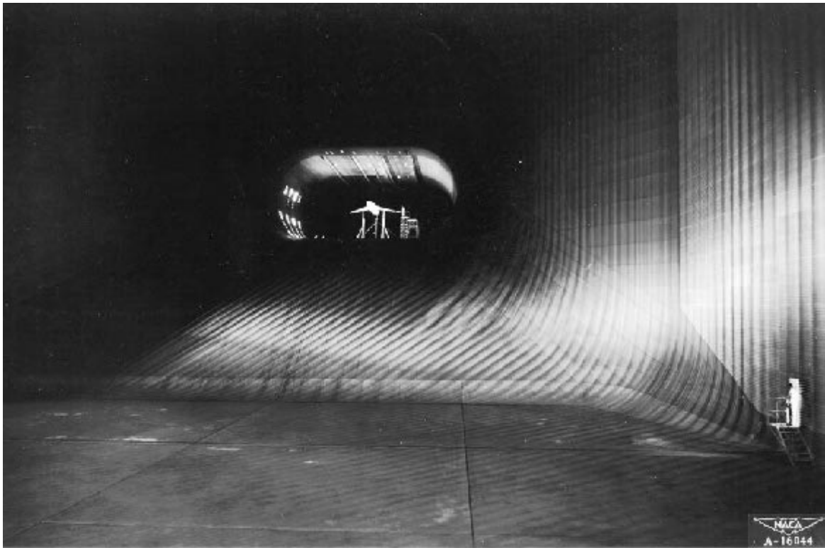
wind tunnel Looking down the throat of the 40- × 80-ft wind tunnel at NASA Ames Research Center. NASA
