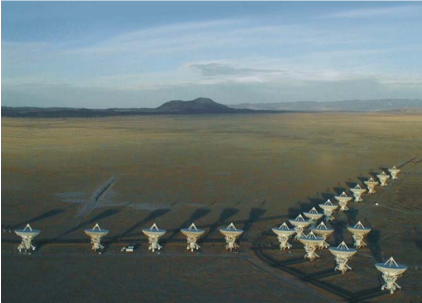
FIG. 1.11 Very Large Array Each of the 27 radio telescopes of the Very Large Array, abbreviated VLA, measures 25 meters in diameter, or about the size of house, and weighs 235 tons ( 2.35 \times 10^5 kilograms). These telescopes are placed along the arms of a Y-shaped array on a desert near Socorro, New Mexico, and interconnected electronically to provide a total of 351 pairs of telescopes. The telescopes can be rolled along tracks to change their configuration and create a radio zoom lens. When the telescopes are pushed to the outer ends of each arm and their output combined in a computer, the VLA creates a radio telescope with a diameter as large as 34 kilometers and an angular resolution that can be smaller than 1 second of arc. (Courtesy of NRAO, AUI and NSF.)
