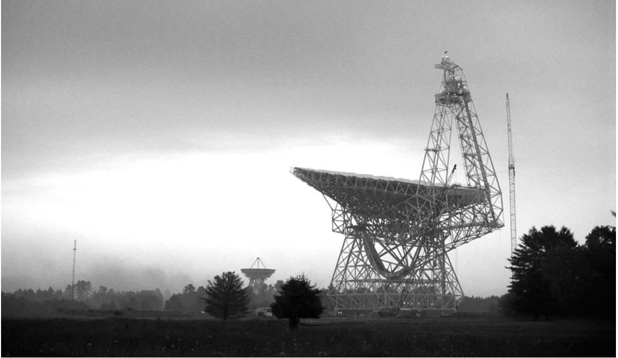
Fig. 3.25. The largest fully steerable radio telescope is in Green Bank, Virginia. Its diameter is 100 \times 110 m. (Photo NRAO)
