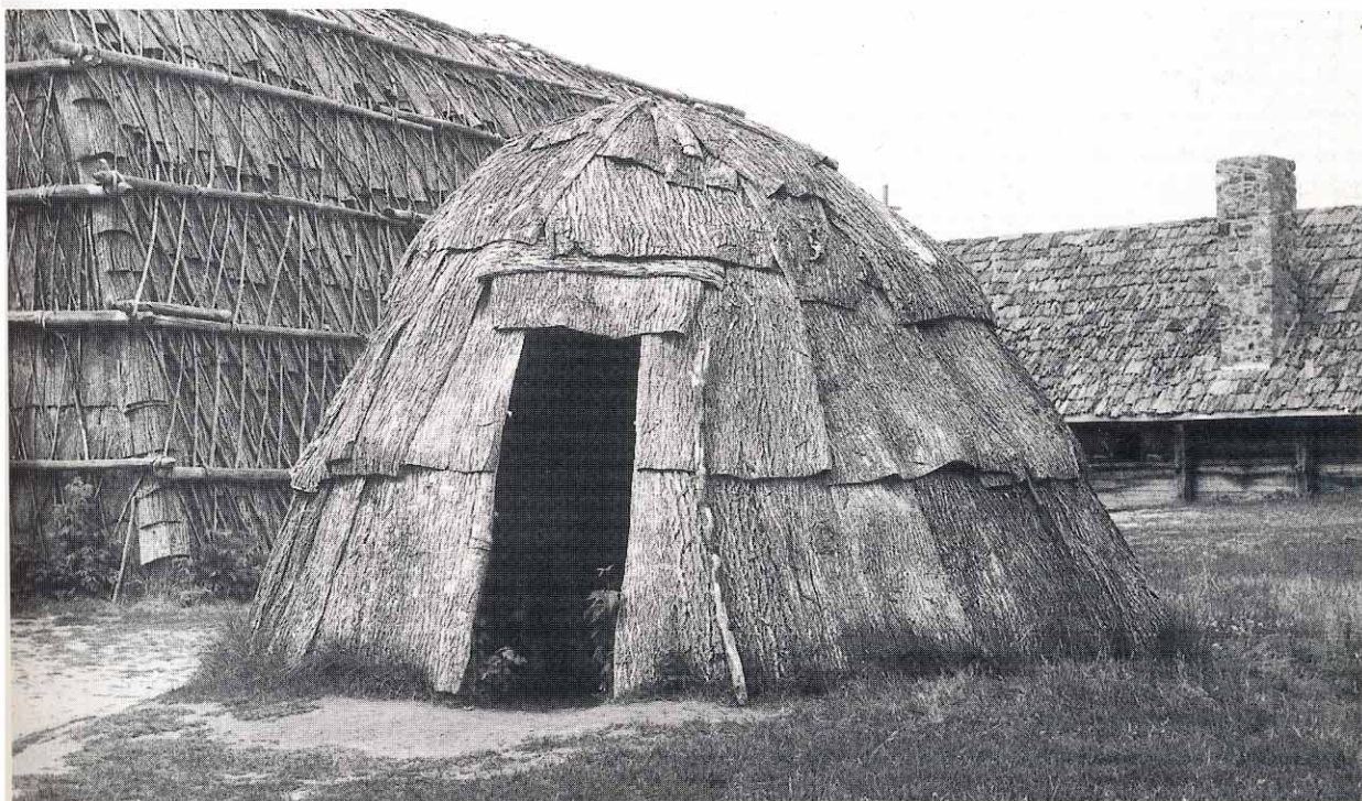
Wigwams of 'classic' shape, constructed of elm bark and poles; and of a squatter conical outline, made of birch bark. (Robin Golden-Hann)
