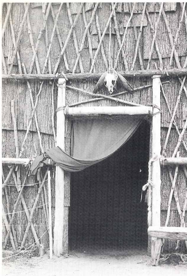
This and the following photographs show reconstructed buildings at St. Marie-Among-the-Hurons, Midland, Ontario, which are based on 17th-century descriptions and archaeological finds. This detail of the doorway of a large elm bark longhouse shows the construction—criss-crossed withies over elm bark sheets. (Robin Golden-Hann)
