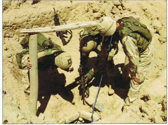
ABOVE LEFT Staff Sgt. Raybon Smith, the Squad Leader for 2nd Squad, 1st Platoon, A Company, 41st Engineer Battalion, uses the flashlight attached to his M4 carbine to light the cave so he and another soldier can set up a third 40lb shaped charge in order to destroy the cave on September 24, 2003. (U.S. Army)
