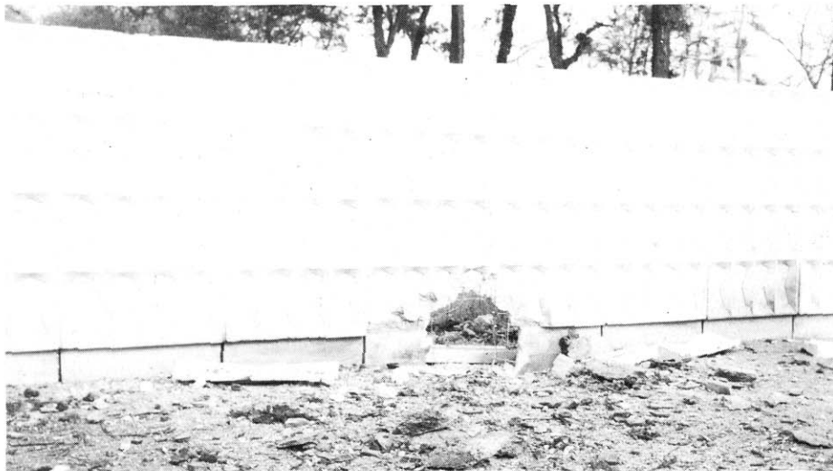
The hole in the embassy wall through which 19 VC entered the compound.
