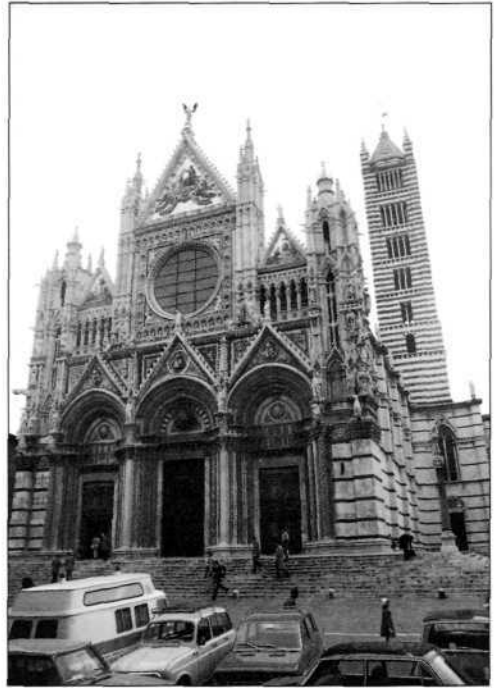
Siena Cathedral is perhaps the biggest and most striking example of the use of black and white horizontal striped masonry as a form of decoration. It almost certainly reflected ideas brought back from the Islamic world and was built between 1196 and the early 14th century. (David Nicolle photograph)
