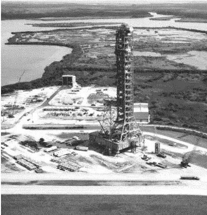
Left: Mobile launcher I was constructed during the period from 1966 to 1968 by NASA at the Kennedy Space Center. It was an integral part of the Apollo program. The structure was altered in the mid-1970s and finally disassembled in 1983 soon after this picture was taken. Right: Earth from 250,000 miles away as photographed by the astronauts of the Apollo 10 space mission in May 1969. [Library of Congress HABS/HAER collection; NASA/Ames Research Center news photo, released.]
