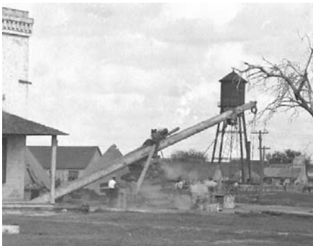
A wireless broadcasting being erected tower at Fort Brown in September 1914. Middle and Right: The erected wireless tower with men on the mast. [Library of Congress South Texas Border Collection of the Robert Runyon Photograph Collection, copyrights expired by date.]
