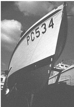
Left: A 110-foot Patrol Coastal (PC) submarine harrier in the construction yard in Stamford, Connecticut, March 1942. The responsibilities of the Patrol Coastal and Patrol Sub Chaser (PCS) vessels were to patrol various waterways and to conduct interdiction surveillance. Right: Current patrol ships like this Cyclone-class Patrol Coastal also provide support to Navy SEAL operations. [Library of Congress FS/OWI photo by Howard Liberman, U.S. Navy news photo, both public domain.]
