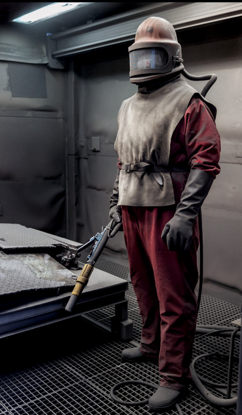
Workers have been taking apart this Soviet-era nuclear power plant, near Greifswald in eastern Germany, since 1995, cleaning radioactive surfaces with steel grit (left) so the metal can be recycled. Germany plans to shut all its reactors by 2022.
