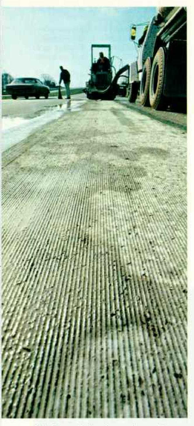
Grinding out the bumps in an old, uneven road requires cutting corduroy-like ridges. A rig pulls 180 12-inch diamond blades used to rehabilitate a much used highway in Georgia. "An impossible job without diamonds," says Jim Parkhurst, job foreman for C. W. Hatcher, Inc., of California.
