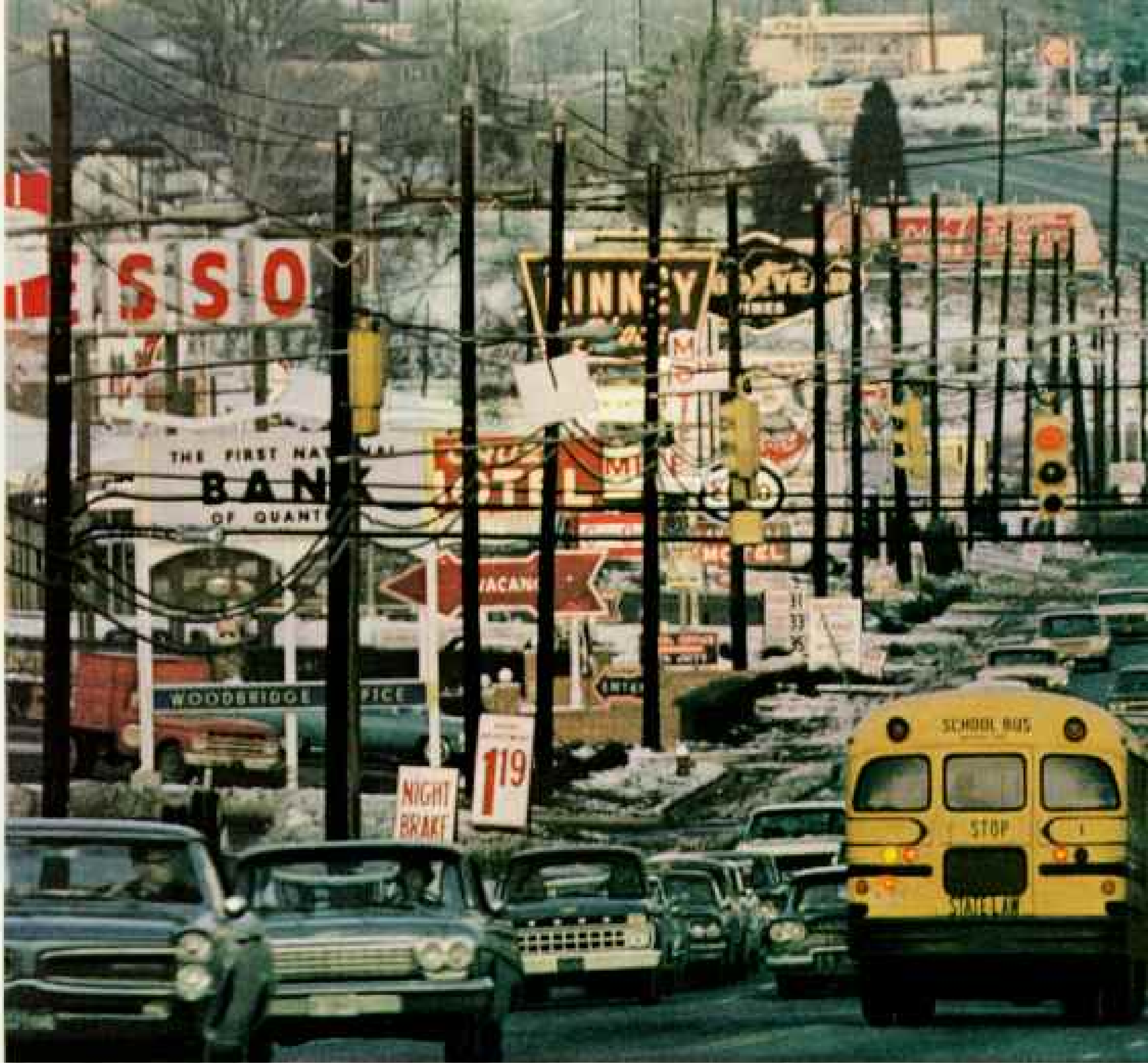
Tangled thicket of traffic hazards confronts drivers on 40-year-old U. S. 1 in Woodbridge, Virginia. There is no median strip to prevent head-on collisions; jumbled signs impair vision; driveways feed autos onto the thoroughfare without warning; narrow shoulders leave little room for human error. The result: a death trap. The old highway follows the route of a
