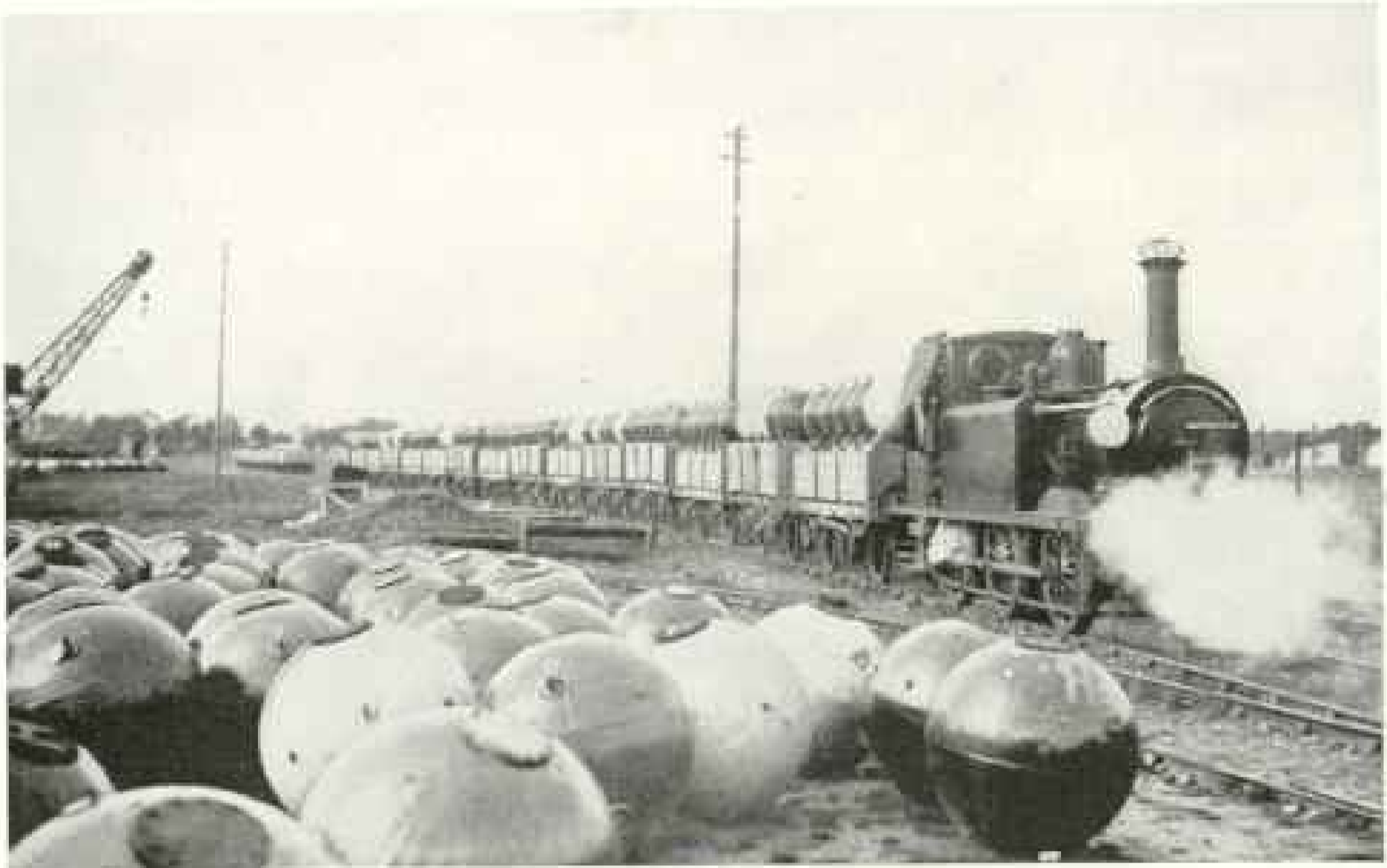
A TRAINLOAD OF AMERICAN MINES PROCEEDING TO THE EMBARKING QUAY The big steel bubbles strewn about in the foreground are each filled with 300 pounds of TNT, one of the most powerful explosives used during the world war.
