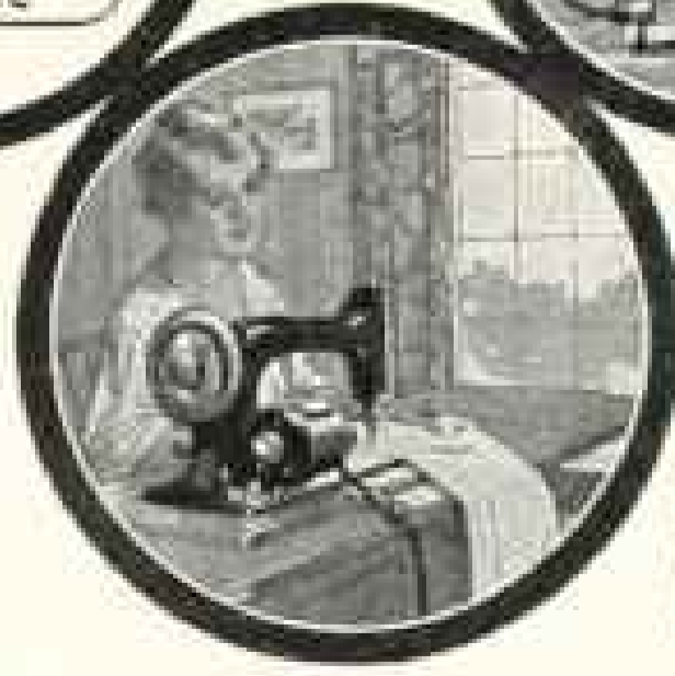
A Westinghouse Sew-Motor makes an electric machine of any ordinary sewing-machine, abolishing the toil of treadling.
