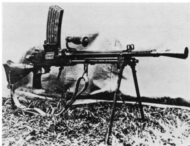
The later and more sophisticated Model 99 weapon of 1939. The box magazine held thirty rounds of 7.7 mm. ammunition. Note the monopod pivoted on the heel of the butt. (Imperial War Museum)
