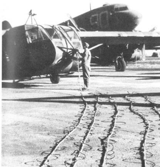
Here a ground crewman double-checks the towrope release on a Waco CG-4A glider. The ropes are laid out in an 'S' pattern to pay out smoothly as the tug takes off. The telephone intercom wire linking the pilots of the glider and its C-47 tug can be seen taped to the towrope in a manner that allowed for rope stretch.
