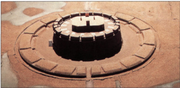
ABOVE Fort Paté: the purest form of a Vauban coast defence battery, built in the middle of the Gironde estuary with a central 'medieval tower' for accommodation and elevated gun positions, surrounded by a lower tier of embrasures for heavier cannon (in theory a total of 30 guns were mounted). Fire could be delivered to all points of the compass, supporting other, larger, fortifications on each bank of the river, thereby blocking access to the city of Bordeaux. The whole thing was built on a shifting sandbank and required two layers of timber to be immersed in the water for a year before building could begin. Note that it conforms to absolutely none of the supposed 'three systems' conventionally attributed to Vauban's art. (Christian Carlet at the Musée des Plans Reliefs)
