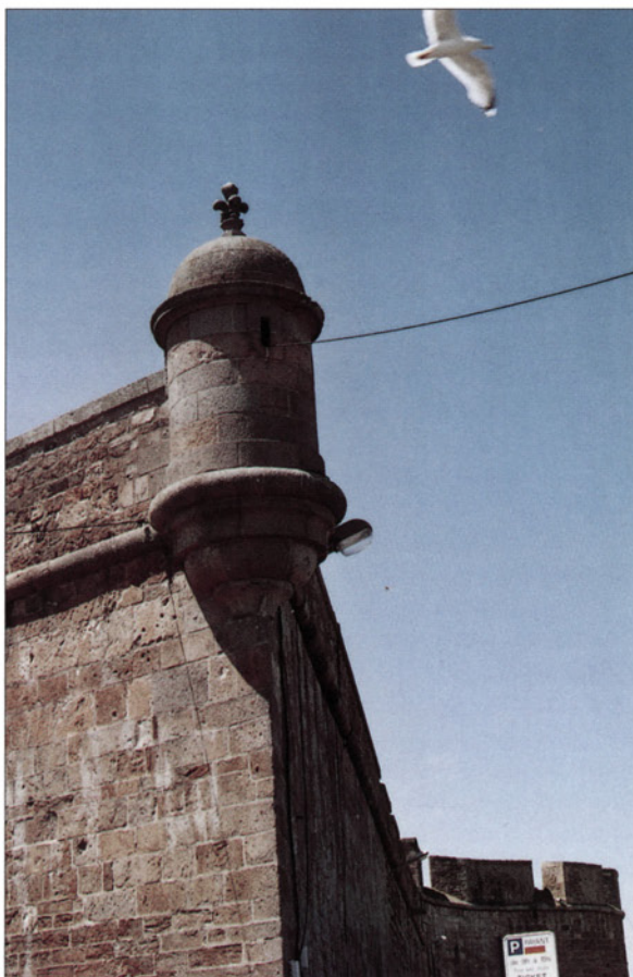
BELOW Masonry sentry box ( echangnette or guérite ) at the angle of a bastion in Vauban's town enceinte at St Malo. (Paddy Griffith)
