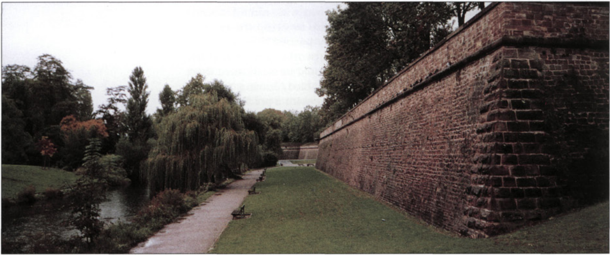
ABOVE The angle of a sandstone bastion at Strasbourg with its flanking bastion in the distance, and a recently landscaped wet ditch to its front. In 1681 the French occupied the city and its enceinte , which had 16 bastions, after which Vauban and Tarade added a bastioned citadel and extensive new water features. (Viv Haywood)
