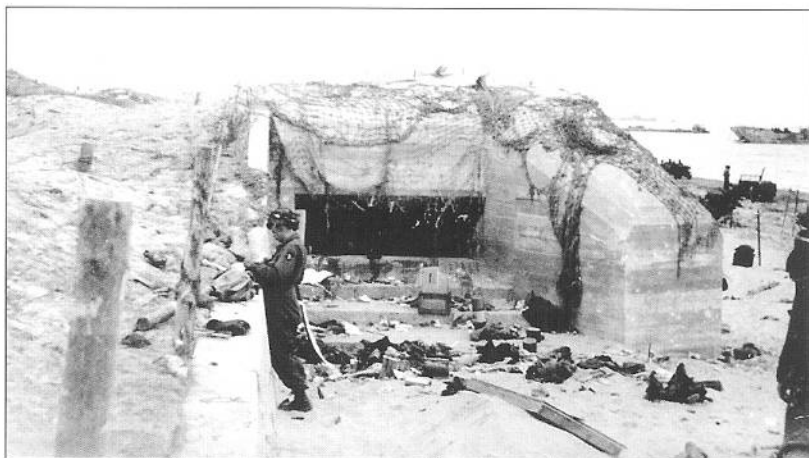
One of the principal elements of the W5 (WN104) strongpoint at Utah Beach was this H667 enfilade-fire casemate for a 50mm gun. Normally, the embrasure would be shielded by a camouflage net to hide its function. (NARA)
