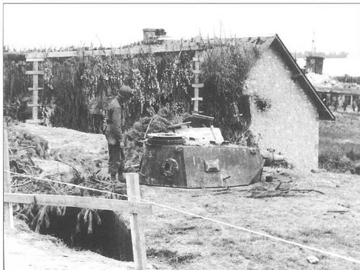
Another example of one of the VK.3001 Panzerstellung , located at the WN68 strongpoint covering the Saint Laurent draw. (NARA)
