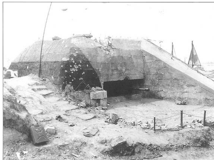
This 50mm anti-tank gun in an H667 casemate proved to be one of the most effective elements of the WN65 strongpoint covering the E-I St. Laurent draw. It was finally silenced by 37mm automatic cannon fire from a pair of M15A1 multiple gun motor carriage half-tracks of the 467th AAA Battalion. (NARA)
