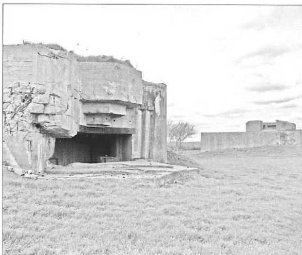
The Azeville battery contained four 105mm gun casemates including these two H650 casemates on the north side of the battery. The casemate in the background was a modified design with a 37mm Flak position mounted on the roof. During a gun duel with the USS Nevada , the gun in the casemate to the right was knocked out by a direct hit. (Author)
