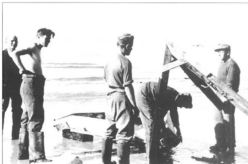
German troops install a steel tetrahedron along the Normandy shore in the spring of 1944. These were usually secured by concrete anchors. (MHI)
