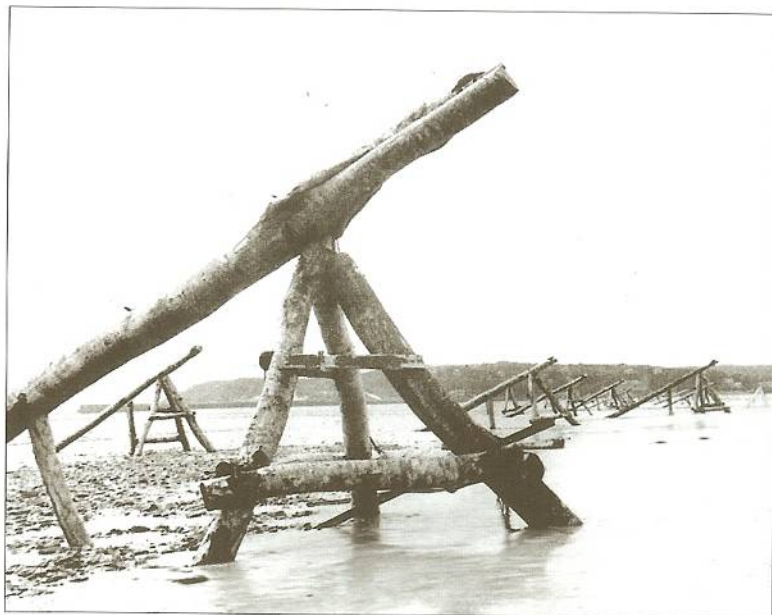
Hemmbalk were a more substantial obstacle developed in the spring of 1944 when it became evident that the simpler stakes were not effective against an on-rushing landing craft. They were usually topped with a Teller mine to blow a hole in the hull of the landing craft. (MHI)
