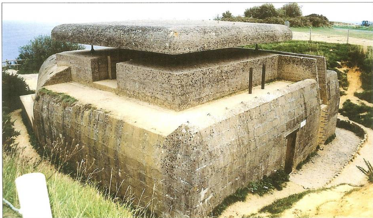
The M262a fire-control bunker of the Longues-sur-Mer battery was the most modern on the Normandy beaches, the only one with an automated plotting and electric data distribution system. (Gary Edmundson)
