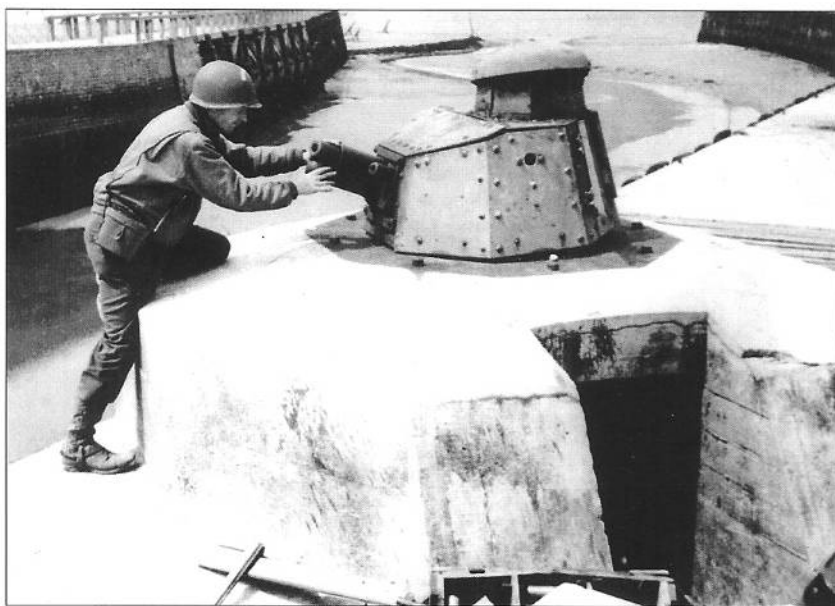
Tank turrets mounted on tobruks were a common feature of the Normandy defenses and this example of a "U" pattern tobruk with World War I Renault FT tank turret was located near one of the breakwaters in Grandcamp harbor between Utah and Omaha Beach. (NARA)
