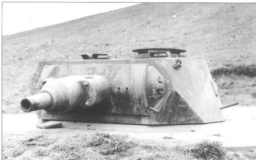
One of the rarer defensive features at Omaha Beach was this VK.3001 tank turret on an H246 bunker, part of WN68. Krupp only completed six of these prototype tanks and their turrets were later released for fortification purposes. A further six new-production T.3001 turrets were built later, four ending up on the Atlantic Wall and two on the Westwall. (NARA)
