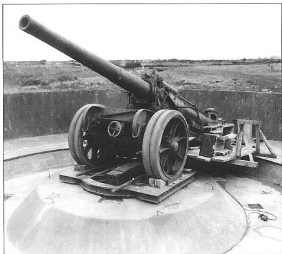
ABOVE LEFT This provides a good example of the type of kettle emplacements first built along the Normandy coast, in this case one of the six 155mm K420(f) gun emplacements at StP 152 near Gatteville. This type of emplacement is patterned after the World War I style, and appropriately enough the gun seen here is a captured French St. Chamond Modele 1916, a type widely used in Normandy due to its excellent 21km range. (NARA)
