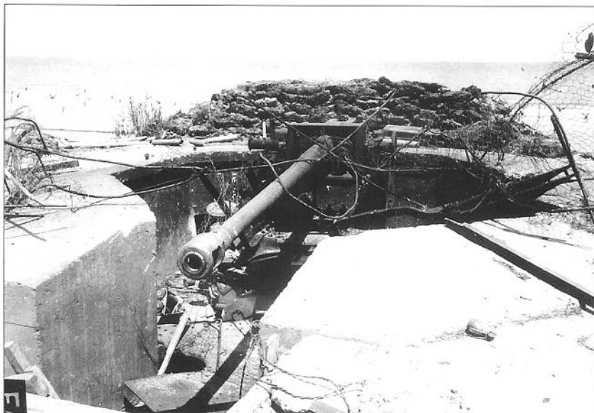
A good example of the common Vf600e open gun emplacement from the strongpoint near Fort Foucarville in the Utah Beach sector. This one is armed with a 50mm pedestal gun with its usual shield blown off during the fighting and lying inside the gun-pit. These emplacements were frequently covered with camouflage and a wire camouflage cage can be seen to the right. The emplacement has been given modest protection from naval fire by a sandbag wall. (NARA)
