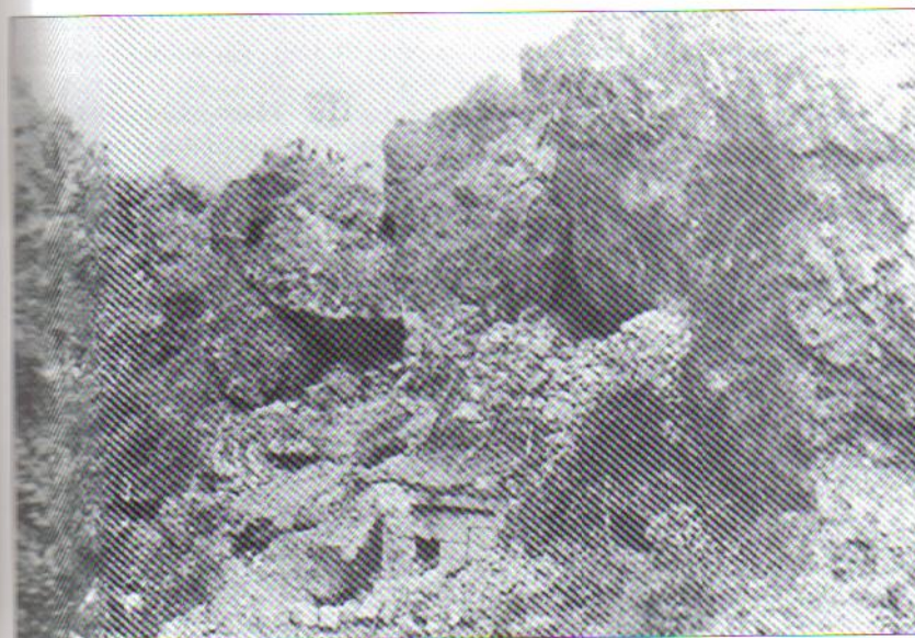
Southern Okinawa, June 1945. Multiple cave openings and firing ports dug into a defended pinnacle were exposed by blasting away the vegetation with direct artillery fire. Most of the openings were protected by piled rock walls, some of which partly collapsed.
