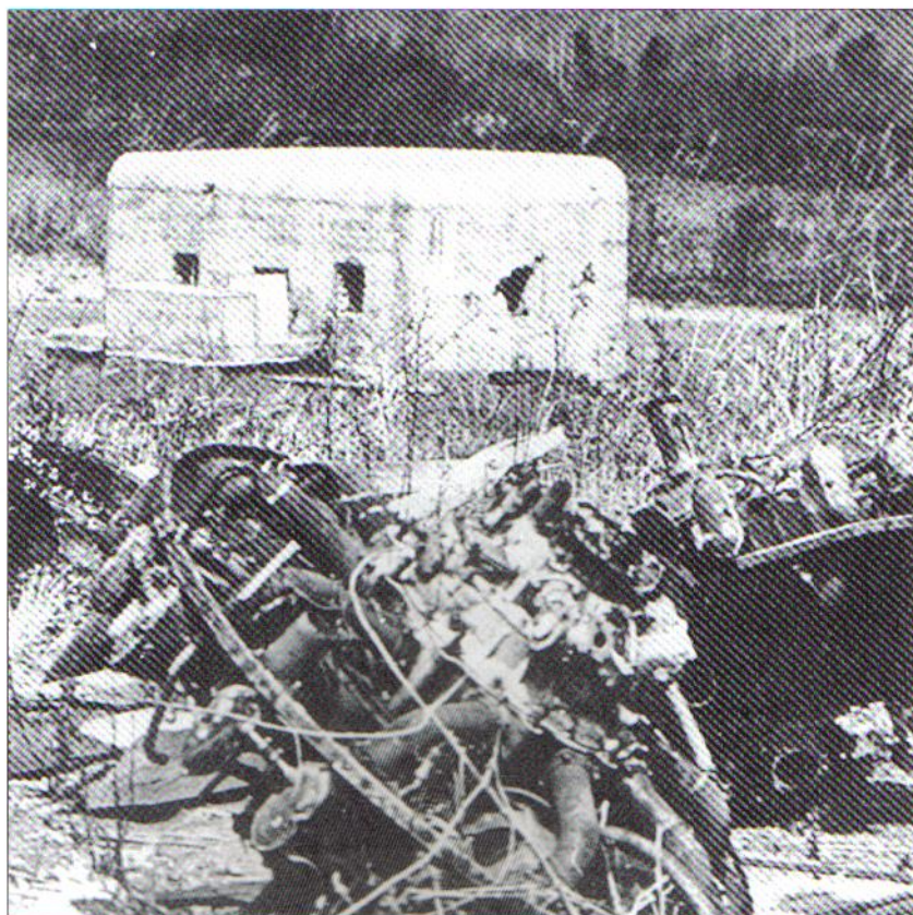
Concrete blockhouses such as this one on Saipan were used for command posts, radio stations, and to shelter various support facilities. Often little effort was made to camouflage them as they were purely bomb shelters and not intended as fighting positions.
