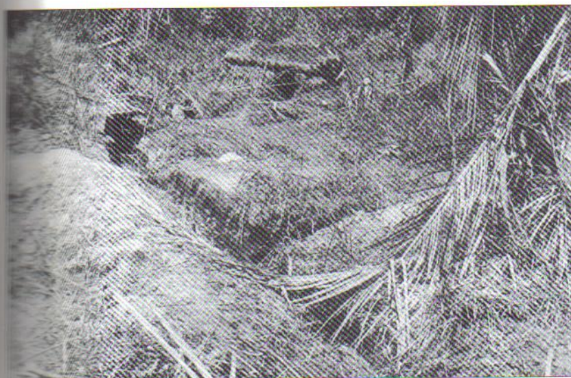
Narrow communications trenches on New Guinea connect pillboxes, one can just be seen in the background. Such small trenches, often covered with palm fronds, were difficult to detect from the ground and air.
