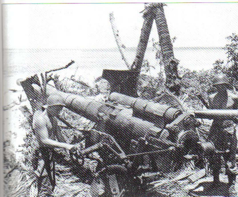
Soldiers examine an IJN 120mm Model 3 (1914) coast defense gun knocked out by a destroyer on Hauwei Island, Admiralty Group. Such gun positions were often a simple circular pit dug in the sand, often without interior revetting. Most coast defense guns were originally designed to be mounted on ships. They retained their steel pedestal mount and were fitted to heavy timber and concrete platforms for shore duty.
