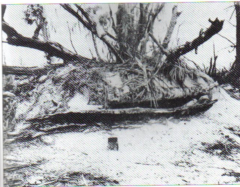
This machine gun pillbox is provided with a rough-appearing firing port, but was difficult to detect from the ground. Built beneath a tree, it was virtually impossible to detect from the air. Camouflaging palm fronds had been pulled away so that the position could be photographed.
