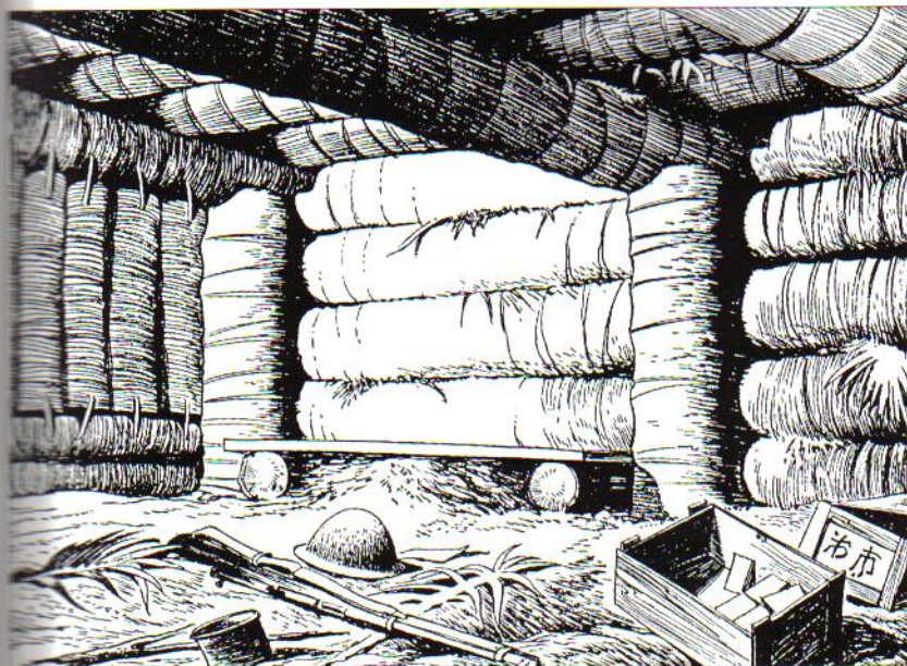
The interior of this bunker provides examples of vertical support posts, log side revetments, and roof support stringers. Steel staples were used to fasten revetting logs together.
