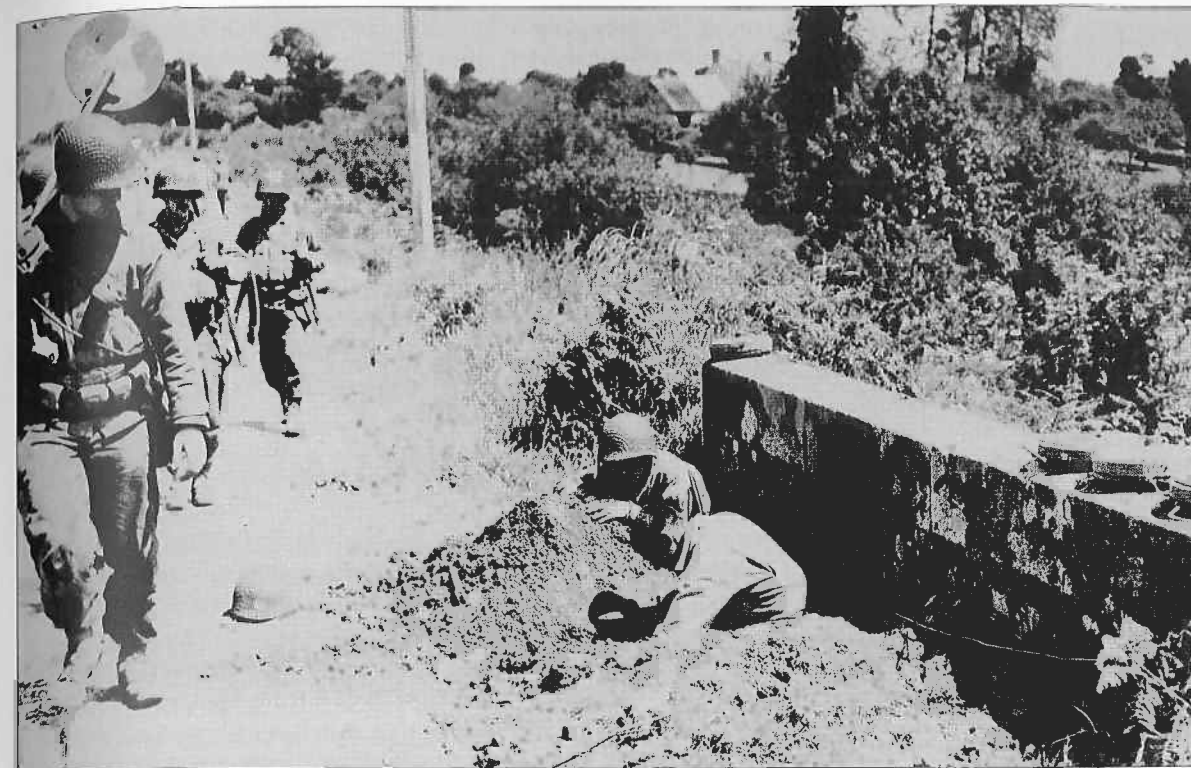
US combat engineers, one carrying an SCR-625 mine-detector, pass others de-mining a roadside at La Haye du Puits, Normandy, on 11 July 1944. Note the platter-shaped German Tellerminen AT mines ( Teller means platter) already lifted and placed on the wall. Much more dangerous to infantry was the 'bouncing bitch' or 'castrator' – the Schrapnellminen 35 or 44 bounding anti-personnel mine, called the 'S-mine' by the Allies. Buried with only the fuse exposed and connected to a tripwire, it was difficult to detect among brush and grass; when tripped, an initial charge sent it 3ft-5ft into the air before it detonated, spraying 360 steel ball bearings in all directions. (NARA)
