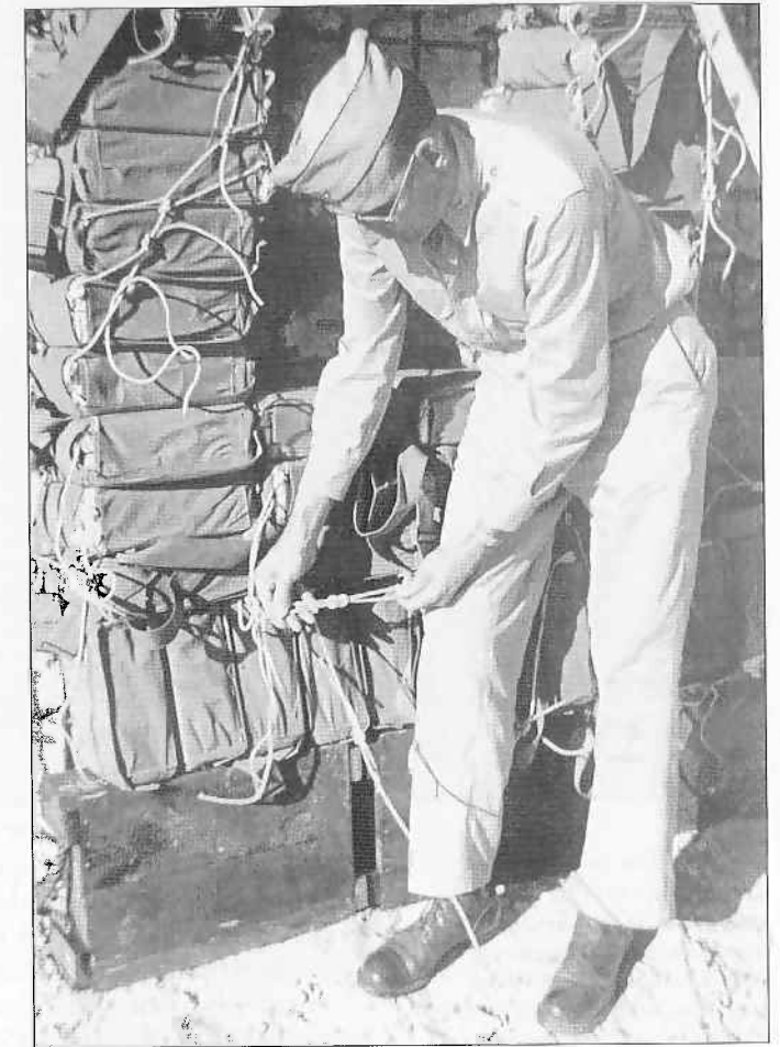
American 22lb satchel charges have been stacked against an AT wall, and the instructor demonstrates how the free ends of each satchel's detcords are linked together by square knots. Extremely heavy demolition charges were necessary to blast a way through AT seawalls facing beaches. One experiment involved stacking 46x 22lb TNT satchel charges in two rows in a wooden rack almost the entire width of the blade of a tank-dozer. The idea was that the tank would lower the blade and leave the rack tipped against the wall; the charges were linked with detcord, so all 920lb of TNT could be detonated simultaneously.
