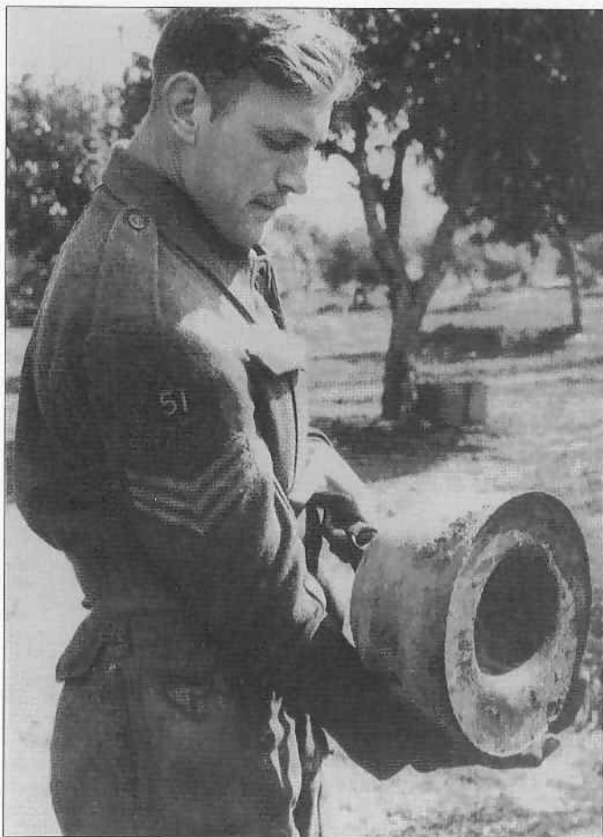
British Royal Engineers sergeant displaying a captured German 12.5kg Hohlladung ('hollow charge'), measuring 11in in diameter by 8.1in high. The dark green sheet metal casing has a detonator well and a web carrying handle at the top. Lacking any 'stand-off' effect, this pre-war munition was soon replaced by the more powerful 13.5kg type with folding legs at the base. (Private collection)
