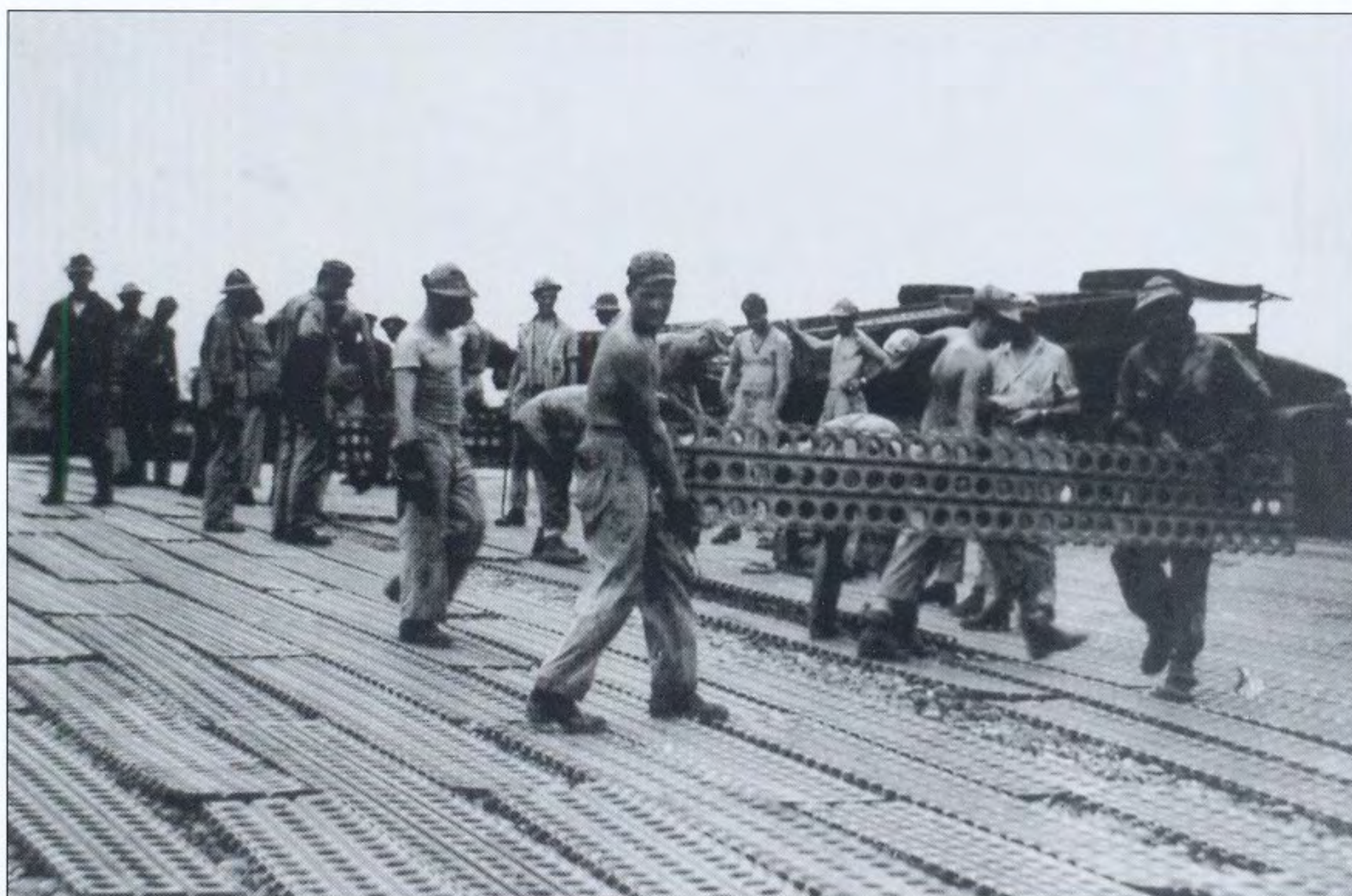
A major Navy contribution to Amphibious Forces were the Naval Construction Battalions (NCB) or “Seabees,” here laying Marsden matting for an airstrip. Well equipped with construction gear, highly skilled and motivated, and famous for their ingenuity, their motto was Construimus Batuimus – “We build, we fight.”
