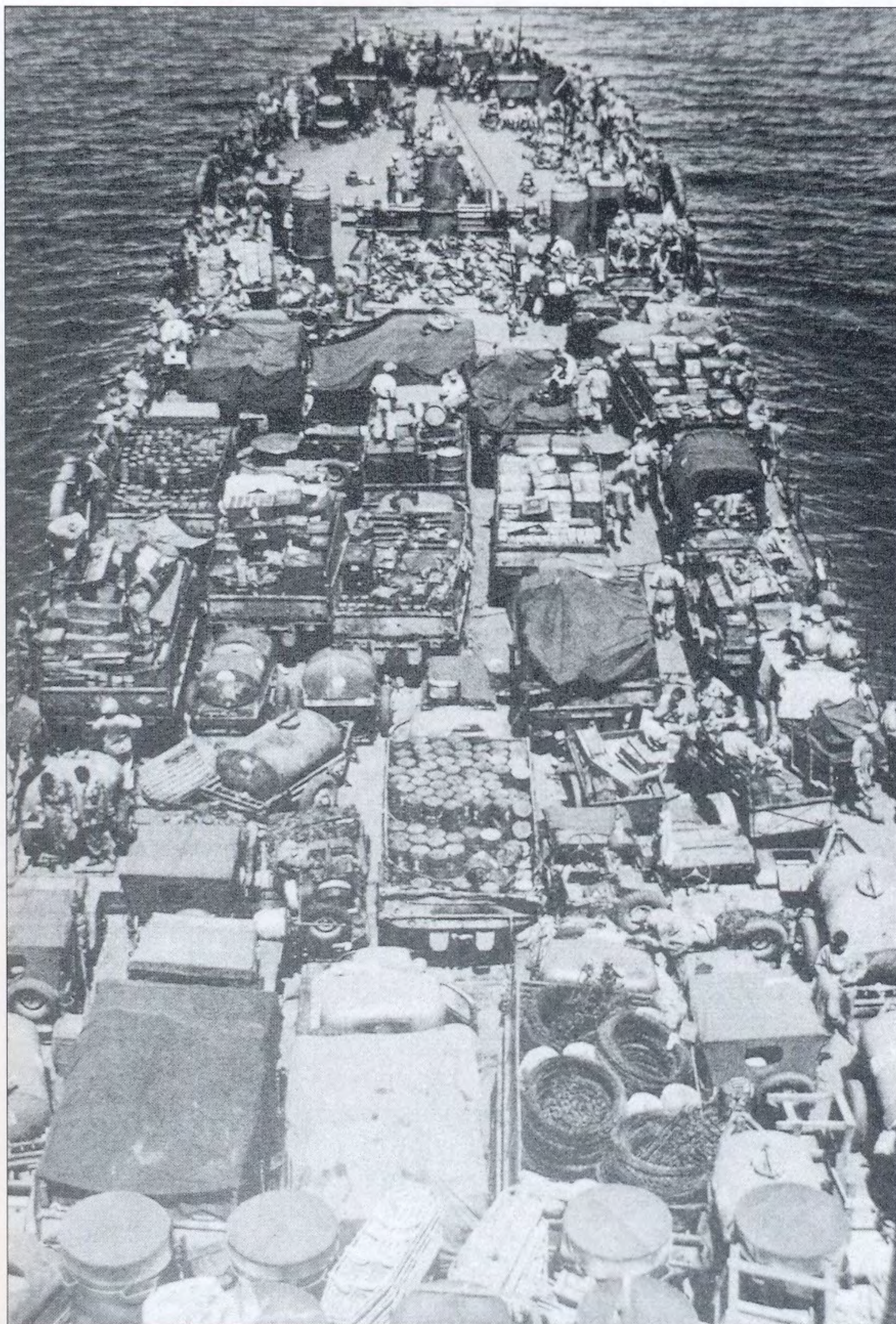
A unit's follow-on echelon embarked aboard an LST en route to Cape Gloucester, New Britain. These trucks loaded with combat supplies and equipment would descend to the tank deck and disembark out the bow doors. The visible gear includes Stokes litters, concertina wire, fuel drums, rations, and 250gal water trailers.
