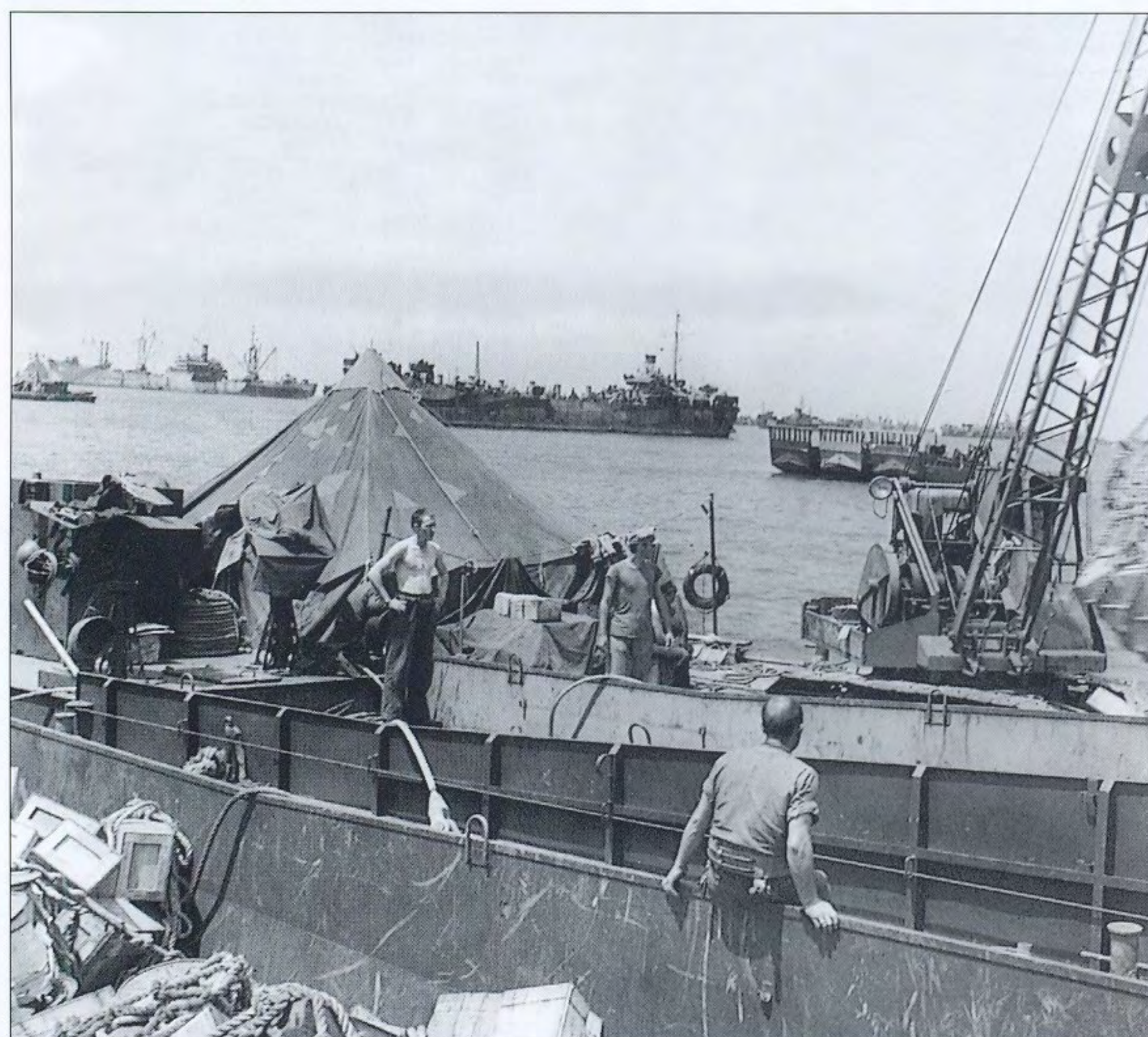
5-ton crawler crane hoisting cargo from an LCM(3) on Okinawa.
