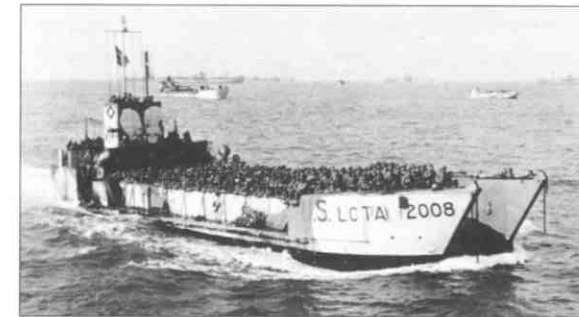
June 1944: men of the 2nd Infantry Division approach the Normandy beaches shortly after D-Day; this LCT (Landing Craft, Tank) was specially designed to carry vehicles directly onto the beach. The USN was slow to master the training of landing units, and in the December 1942 North African operation about 50 per cent of the landing craft were lost due to inept boat handling in choppy water. By 1944 skills had improved considerably; the Navy was able to land over 21,000 troops and 1,700 vehicles over Utah Beach on D-Day alone.
