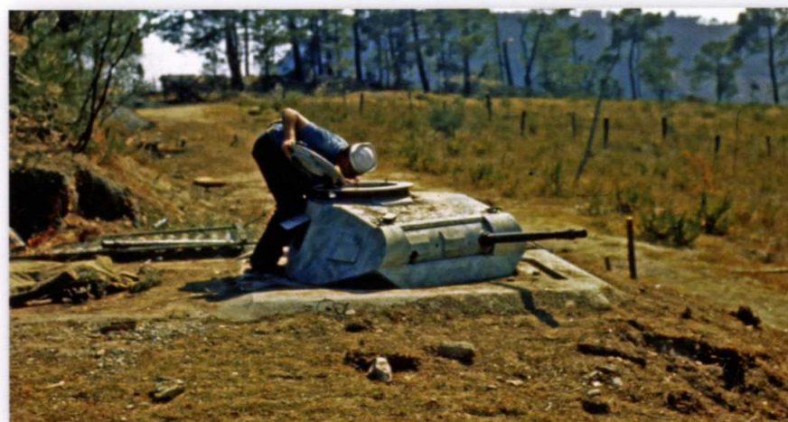
One of the most common defenses on the Var coast was the Panzerturm consisting of the turret from an obsolete tank such as this PzKpfw II mounted on a concrete foundation. (NARA)
