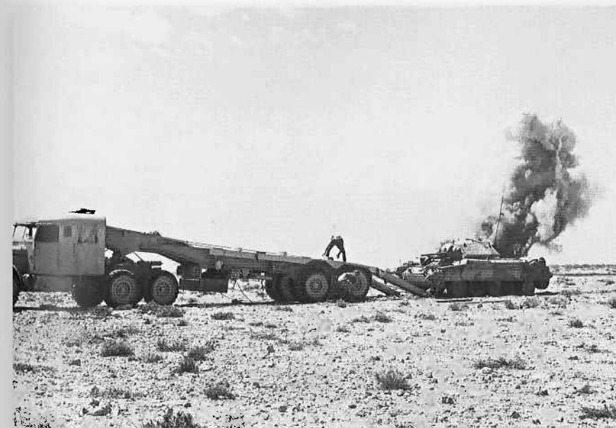
A broken-down or possibly damaged Crusader tank is recovered from the desert and loaded onto a tank transporter to be ferried back to a maintenance centre for refurbishment and subsequent return to battle. (IWM, E13080)
