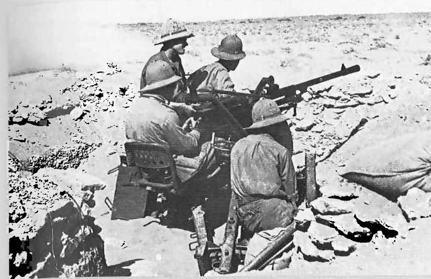
Italian troops man a Breda 20/65 model 35 cannon. This 20mm gun was designed in 1934 as an anti-aircraft weapon, but had a dual role in the desert where it served as an anti-tank gun, albeit with a poor reputation and inferior performance when compared with most other weapons. (IWM, MH5867)
