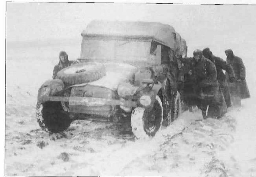
German troops attempting to push a Krupp L2H143 1.5-ton light truck along an icy Russian road. Most German wheeled vehicles did not perform well under these severe conditions. (Nik Cornish)
