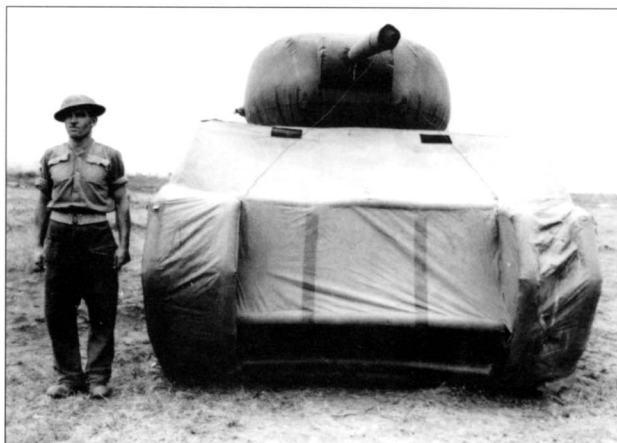
The Allied positions around Anzio were so exposed to German observation from the Alban hills that various methods of deception had to be used to mask troop deployments. This type of inflatable Sherman tank was deployed by British forces to deceive the Germans regarding actual force locations. (NARA)
