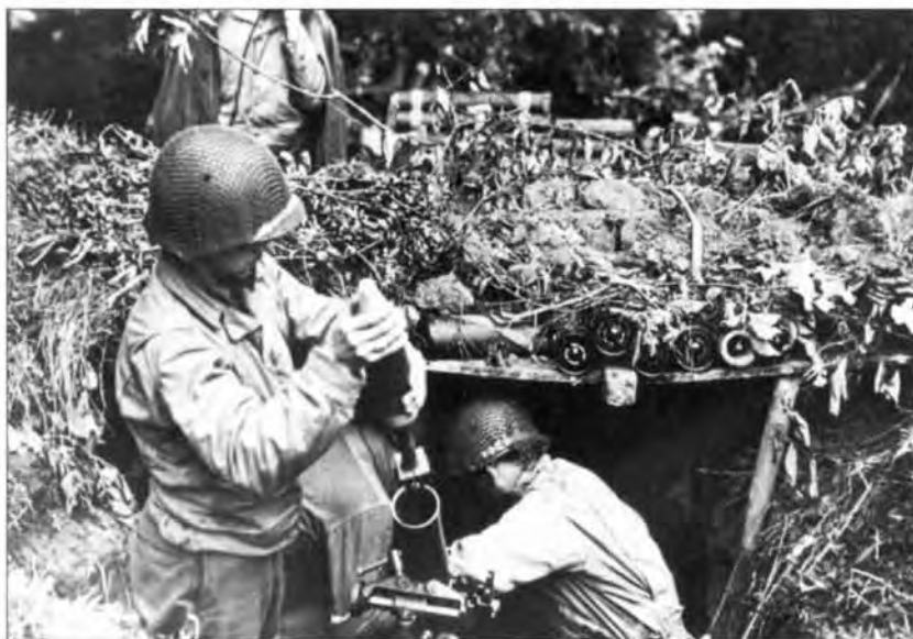
LEFT An American 81mm M1 Mortar firing in support of an infantry attack in Normandy. The mortar had a minimum range of 100 metres, a maximum range of over 3,000 metres and could fire a 3kg bomb. (US National Archives)
