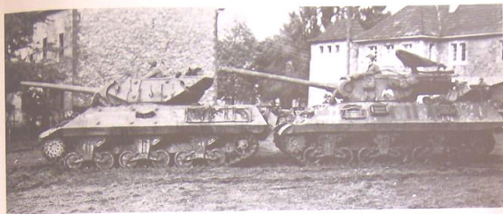
Although the two vehicles were carried on similar suspensions, the M36 (right) can easily be distinguished from the M10 (left) by its larger gun and distinctive turret. (Imp. War Mus.)
