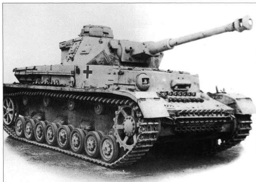
Pz.Kpfw.IV Ausf.G Fgst.Nr. 83072 assembled by Vomag in September 1942. The 7.5 cm Kw.K.40 L/43 was fitted with a double baffle muzzle brake. This tank was captured and sent to England for examination in 1943. The rack for seven spare track links mounted on the glacis was introduced from June 1942. (TTM)
