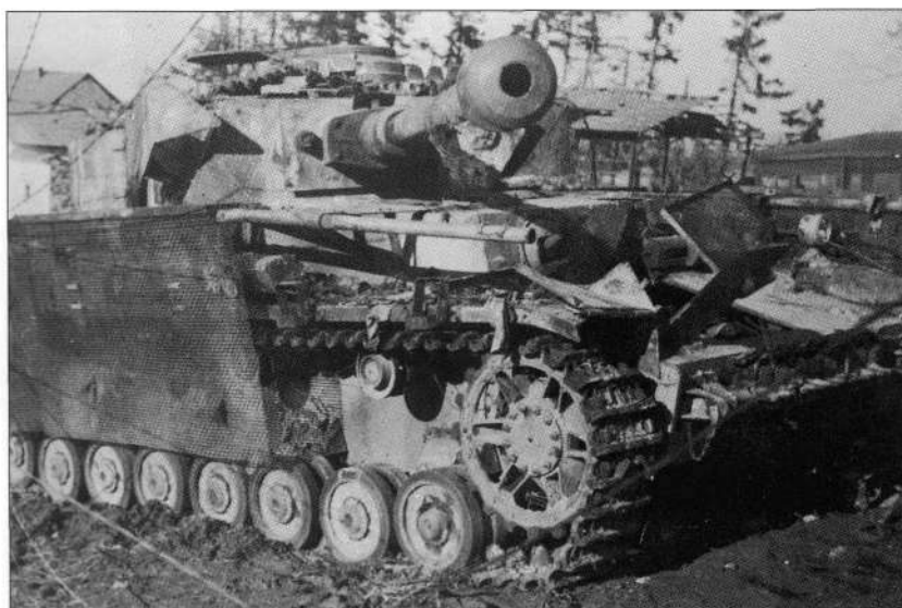
From Pz.Kpfw.IV Ausf.J. Fgst.Nr. 92301 in September 1944 a completely new design of side Schürzen made from wiremesh was introduced. This improved camouflage and the associated rails allowed use of the Schürzen even when the wide Ostketten (tracks for the east front) were fitted. The hatch of the commander's cupola was now modified to pivot to the side. (TTM)
