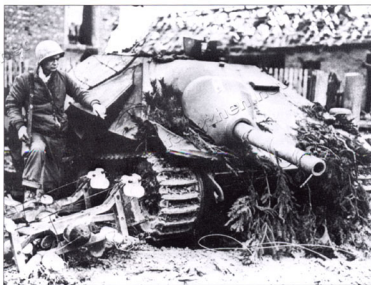
A blown-out Hetzer, evidently caught in a village under bombardment. From the massive fractures in the main armour, it seems to have suffered a direct hit from a large-calibre high explosive shell. (RAC Tank Museum)
