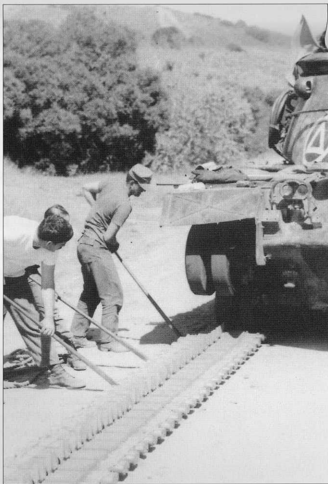
Trainees use pinch bars to align a broken track at the Camp Pendleton tank school. The red warning flag on the tank commander's cupola indicates that the tank is immobilized in the road, and is a crash hazard. (NARA)
