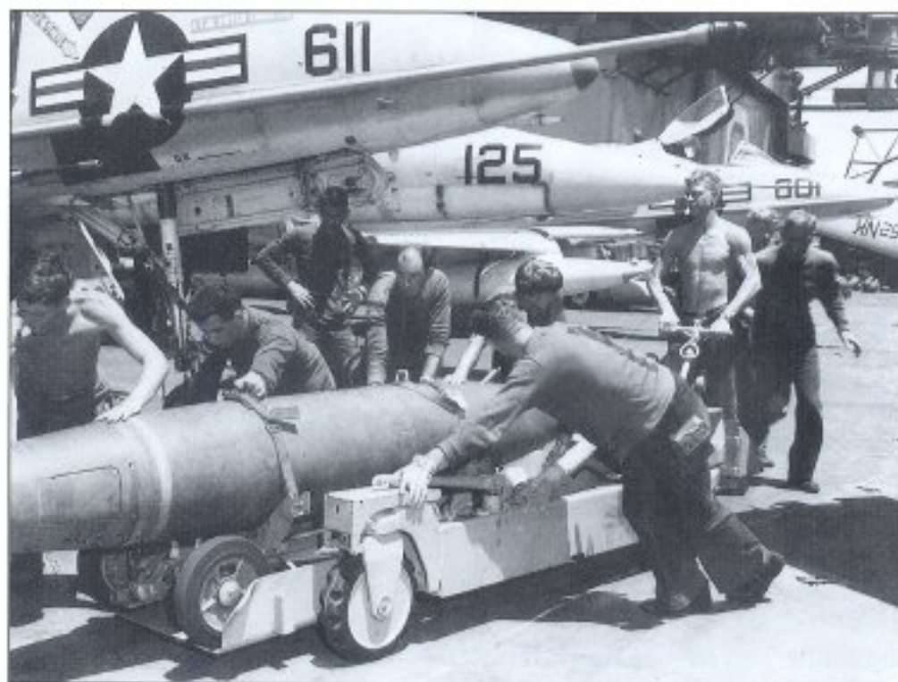
Ranger ordnancemen position a Mk 84 2000-lb bomb in front of an A-4C from VA-146. Note the nose of an RA-5C (Modex 125) from RVAH-9 parked between the two 'Blue Diamonds' jets
