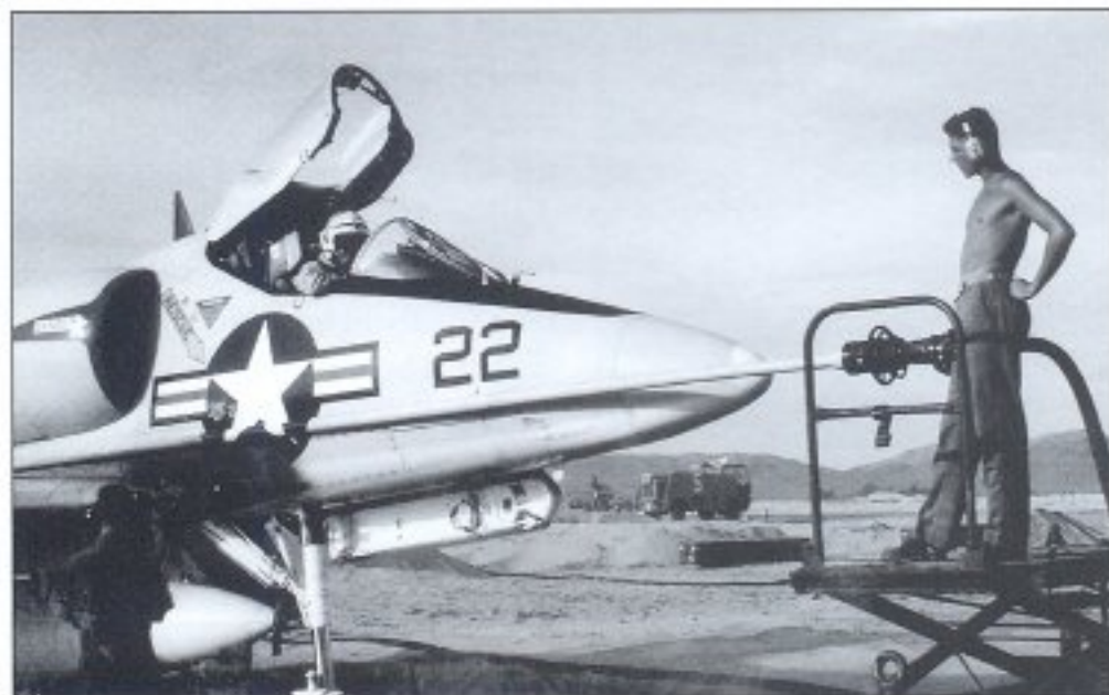
A groundcrewman refuels A-4C BuNo 148465 from VMA-225 through its aerial refuelling probe – a rather unusual, but expedient, method! This aircraft, photographed here in June 1965, was also supplied to the Republic of Singapore Air Force in 1980
