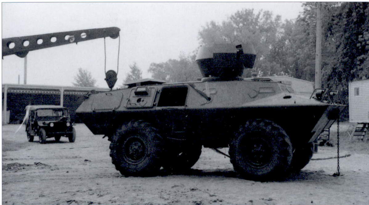
This late V-100 is shown at Rock Island Depot, and is fitted with a 40mm turret. The 40mm turret, which was a modified air cavalry turret, was developed in response to requests by MPs for more firepower for their vehicles. (Copyright Cadillac Gage Textron Inc.)
