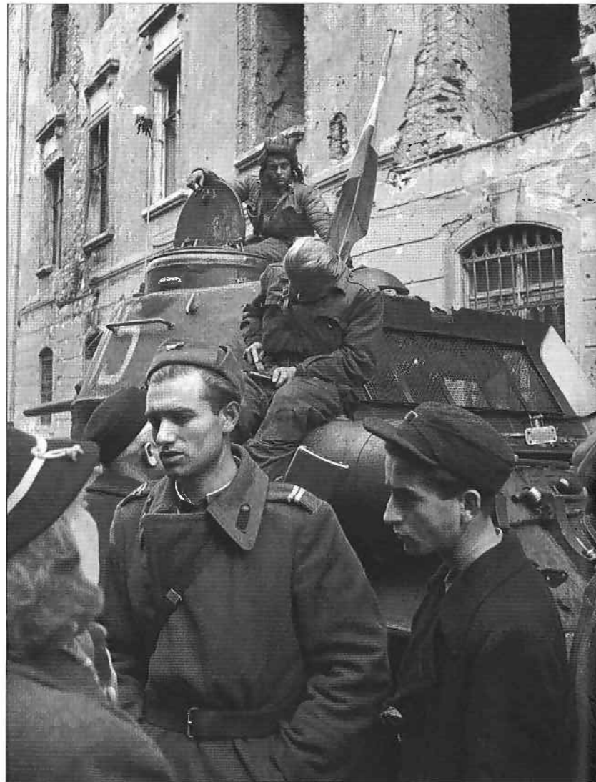
In a street showing war damage, an Army corporal discusses events with Budapest civilians; see Plate E1 commentary for details of typical insignia changes. The T-34/85 crew fly a large Hungarian flag – since both sides used this type, instant identification was crucial. (Lessing Collection No.56-09-12/ 35A)
