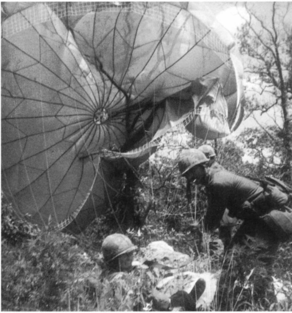
A paratrooper's nightmare, trees and rocks. Members of the 36th Abn. Bde. attempt to untangle a T-10 canopy at Ft Chaffee, Ark., 1977. The anti-inversion netting can be seen on the canopy's skirt, designed to prevent suspension lines from slipping over the canopy. (author's collection)
