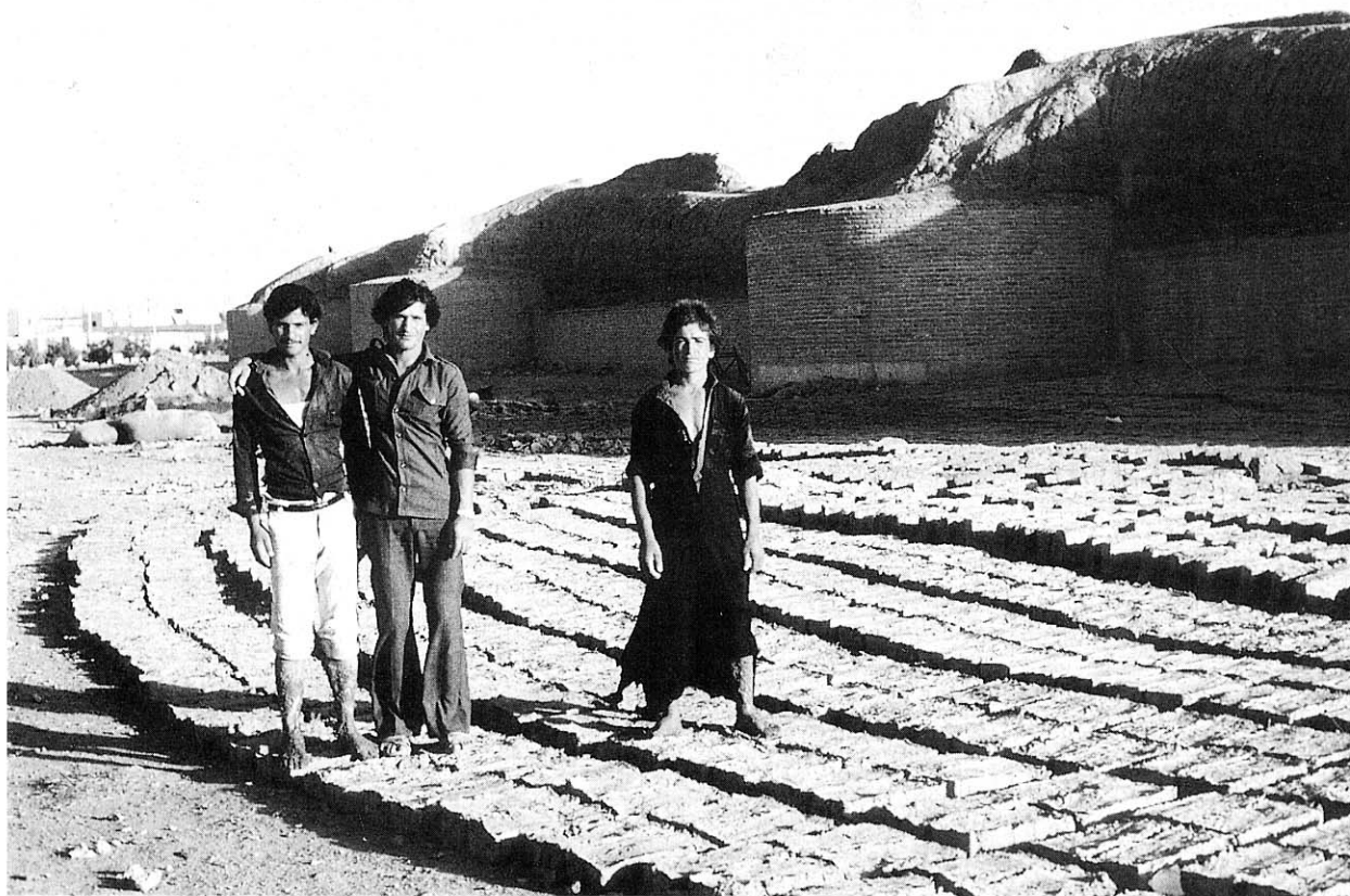
Repairing the Abbasid walls of Raqqa with sun-dried mud bricks as originally used in 772. The massive mud brick core of the wall and solid half-
