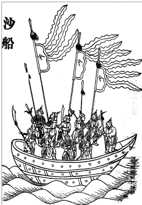
The 'sand boat', a word sometimes used for a Chinese warship, which is shown here crudely drawn and full of armed men. One source says, 'their bottoms are flat and broad; they can sail over shoals and moor near sandbanks, frequenting sandy creeks and havens without getting stuck'.
