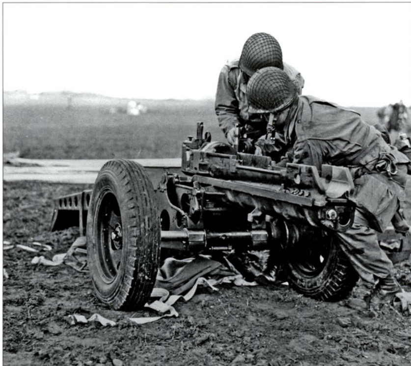
A major problem facing the parachute field artillery was the need to break the 75mm M1A1 pack howitzer into several loads for parachute delivery. This created the risk that key elements would be lost during the airdrop. Here, gunners from the 101st Airborne Division re-assemble a 75mm pack howitzer following a practice jump near Newbury in England on November 23, 1943. (MHI)
