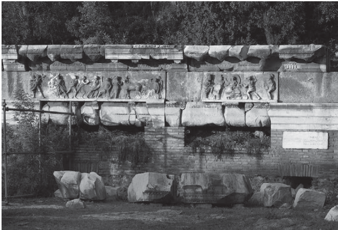
An entablature, or horizontal molding, from the Basilica Aemilia et Fulvia hints at the grandeur of this public building, constructed in 179 BC. Manuel Cohen/Getty Images
