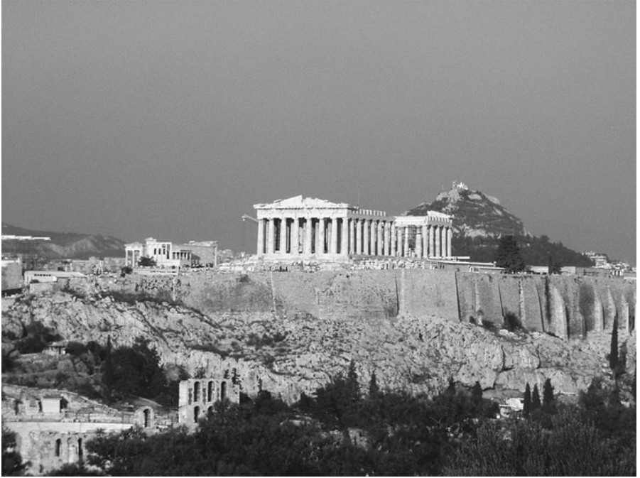
Fig. 6.2: In the mid-fifth century B.C., the Athenians built the very expensive Parthenon temple on their city-state's citadel (the Acropolis) as a second temple honoring their patron goddess Athena and proclaiming their prosperity and military success. The older Athena temple sits to the left of the larger Parthenon in the photo. Wikimedia Commons.
