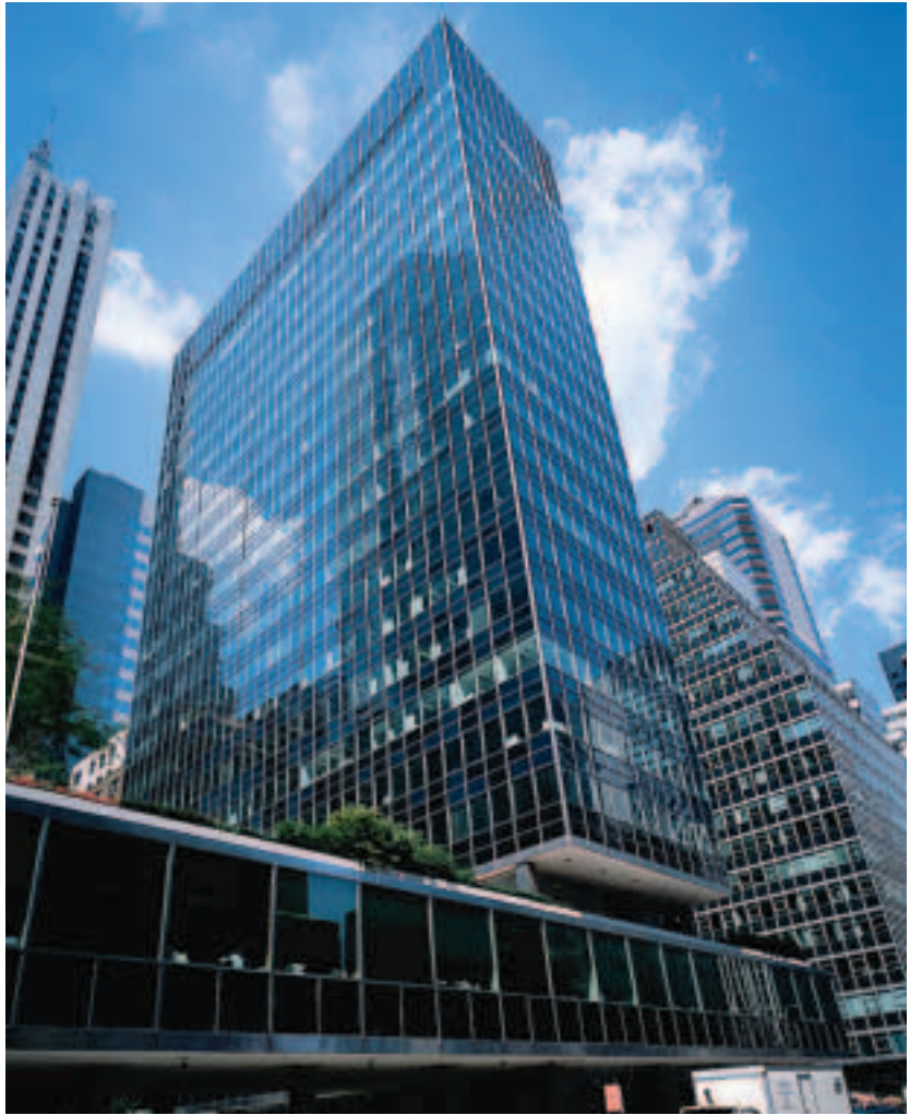
FIGURE 23.30 Notice the steel framework, walls of glass, and absence of ornamental features. How is this building different from the Wainwright Building (Figure 23.29)?
