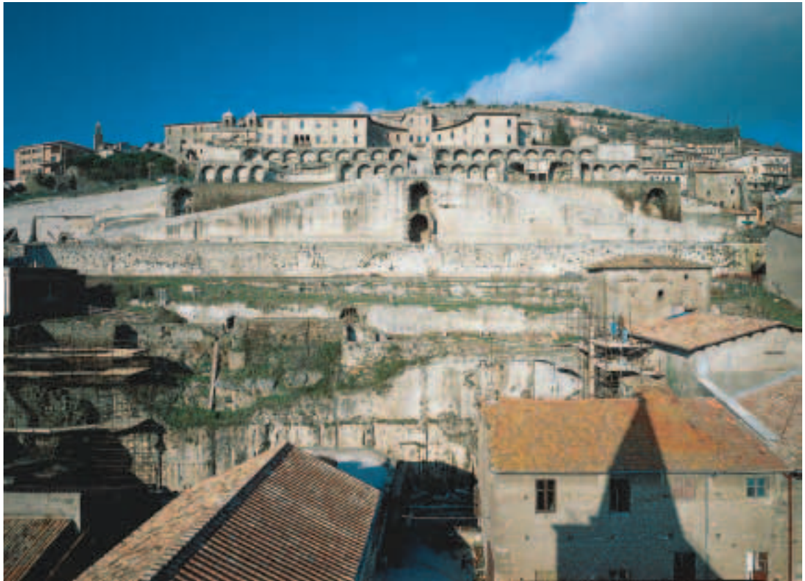
■ FIGURE 9.7 Here Roman builders constructed staircases leading to a series of seven terraces built into a hillside. How does this technique differ from the way Greek builders used a hill site for the Acropolis?
