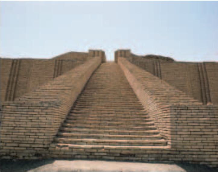
■ FIGURE 6.9 At the center of every Sumerian city-state, a ziggurat stood on a huge platform made from clay reinforced with brick and asphalt. Here, one of three stairways, each with a hundred steps, led to the top of the platform. What role did the ziggurat probably play in the daily lives of the local people?
