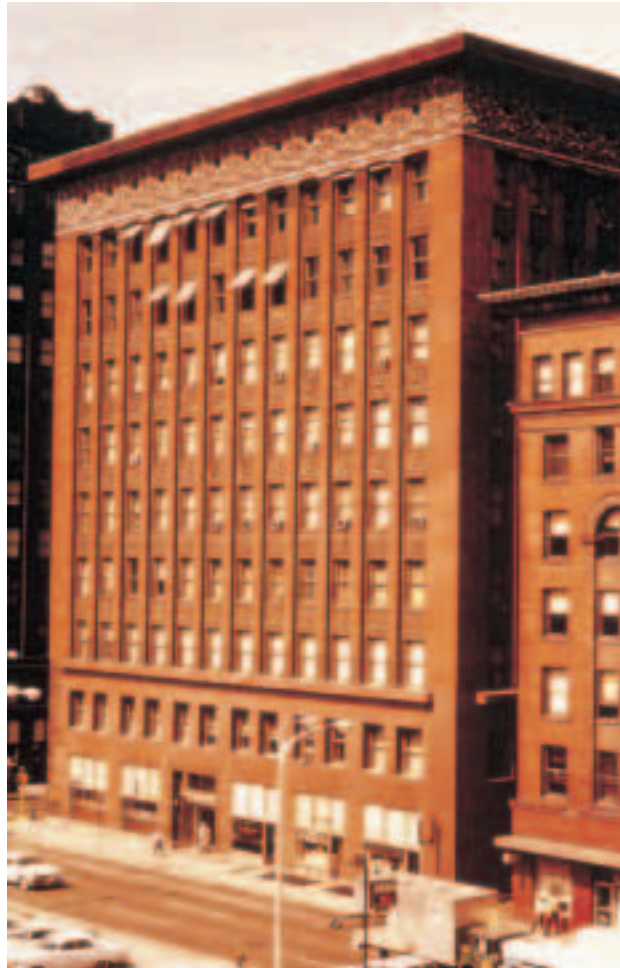
FIGURE 23.29 Vertical steel beams support the walls of this building. What made this building startling when it was constructed? How does it compare to familiar buildings in your community?
