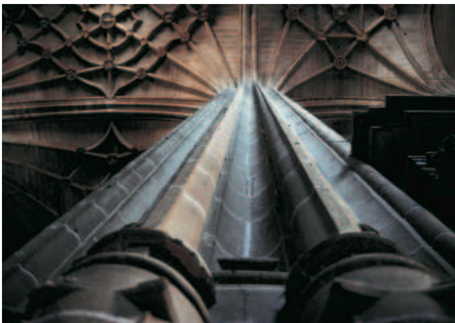
■ FIGURE 15.4 The introduction of pointed arches made it possible to use this kind of slender column or pier inside a large cathedral. In addition to these piers, what else was used to support the heavy stone ceiling of cathedrals?
