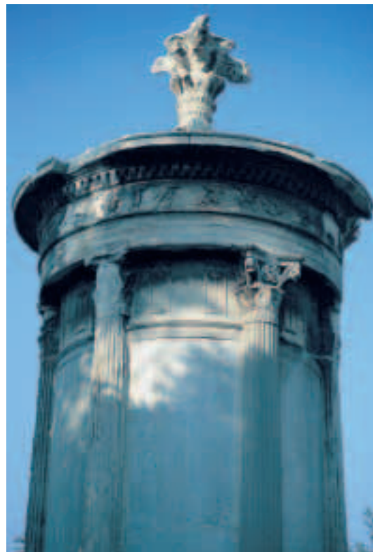
■ FIGURE 8.10 The columns on this monument are the first known example of the Corinthian order on the outside of a building. Describe the form of this structure. How does it differ from the form used for the Temple of Athena Nike (Figure 8.8)?
