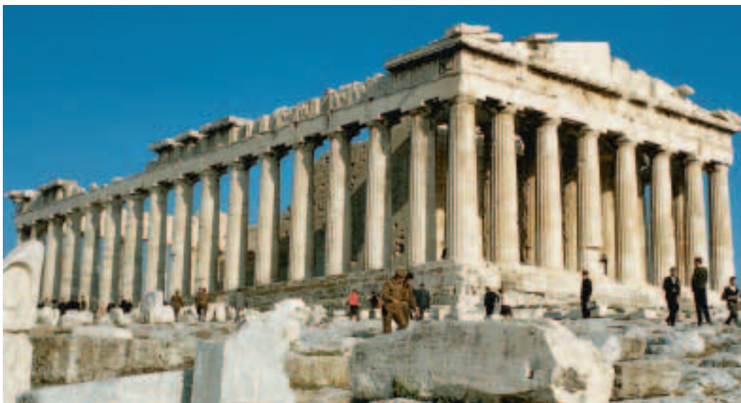
■ FIGURE 8.3 Greek architects used the post-and-lintel method of construction. Identify the posts and lintels in this temple. How would you describe the overall balance of this building? What adjective best describes this temple?
