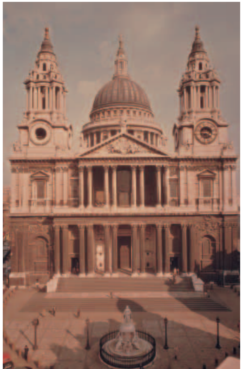
■ FIGURE 20.11 The deep porches on this cathedral create a pattern of light and dark values. What characteristics does this cathedral have in common with classical structures?
