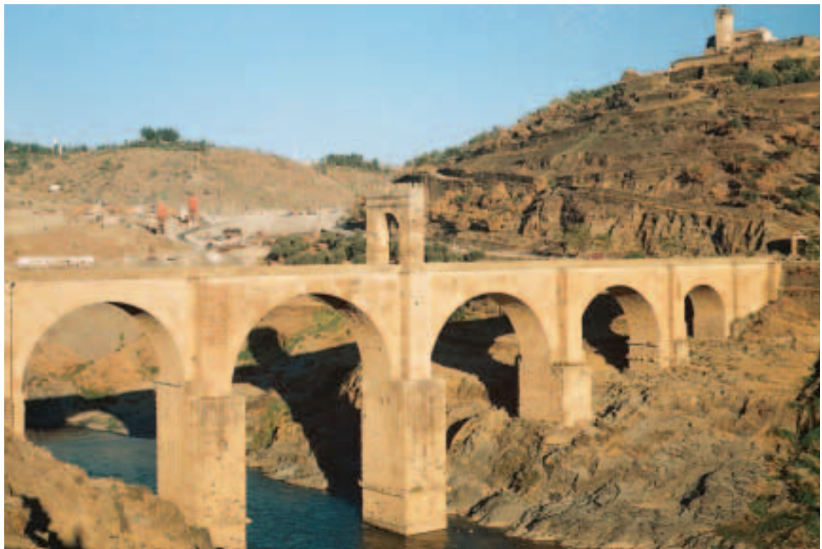
■ FIGURE 9.10 This bridge near Alcantara, in Spain, was built about A.D. 105. It still stands today, providing a way for traffic to cross the river, in the same way it stood nearly 2,000 years ago. What can you conclude about the Romans' introduction of the arch and their use of concrete?
