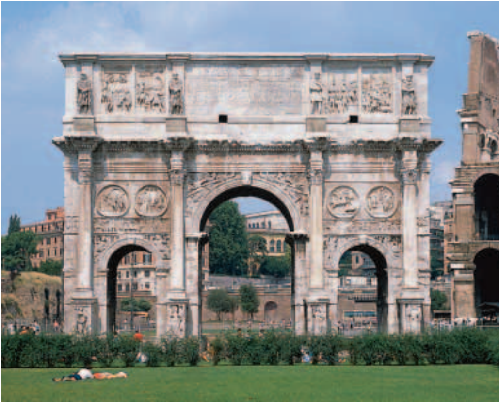
■ FIGURE 9.19 The successful general and his mounted officers would have paraded through the large central arch. The foot soldiers would have marched through the smaller arches on each side. What does this kind of structure indicate about the importance of the army in the Roman Empire?
