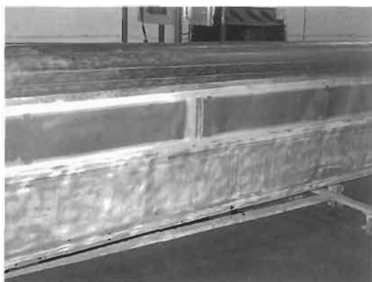
Fig. 39.10. Finished patch.
