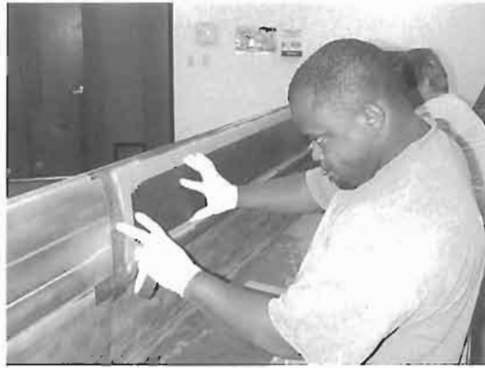
Fig. 39.7. Patch application.
