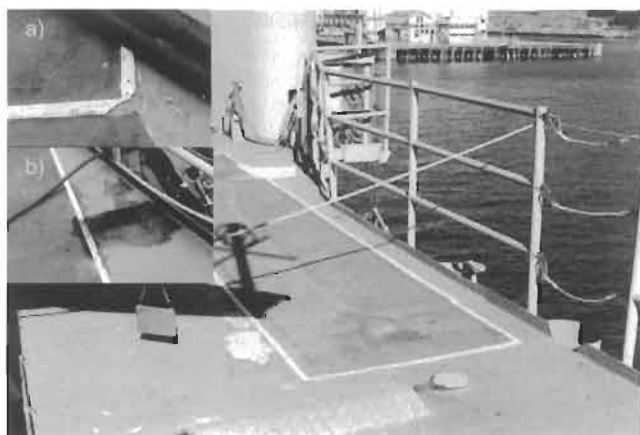
Fig. 42.10. Weathering of composite reinforcement (Starboard side) and typical damage inset (a) and (b).
