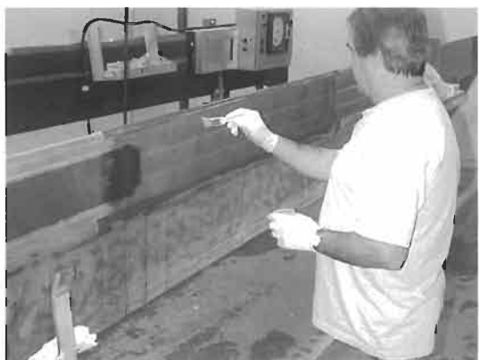
Fig. 39.4. Silane application.
