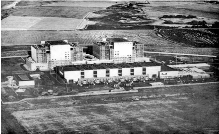
Plate 1.3 A pictorial view of Bradwell nuclear power station (with compliments of CEGB)
