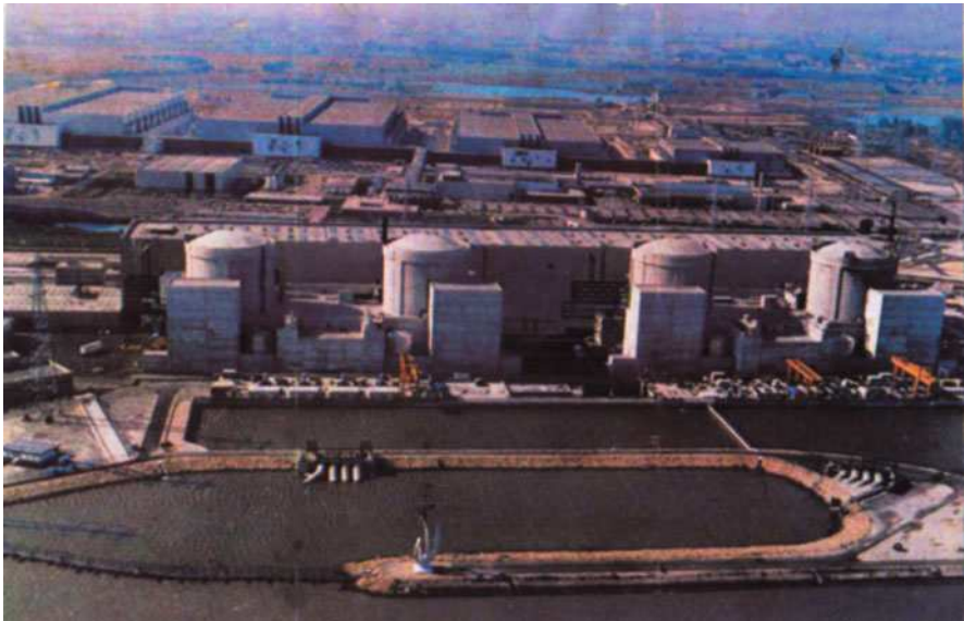
Plate 1.14 Tricastin power station, PWR nuclear power station (Central France)
