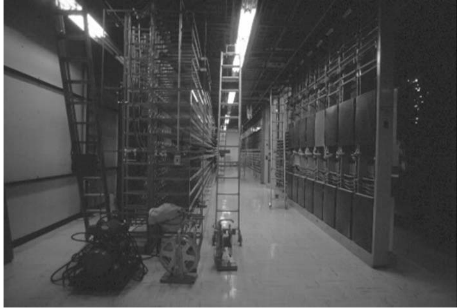
Figure 1-9 Central office and main distribution frame.
